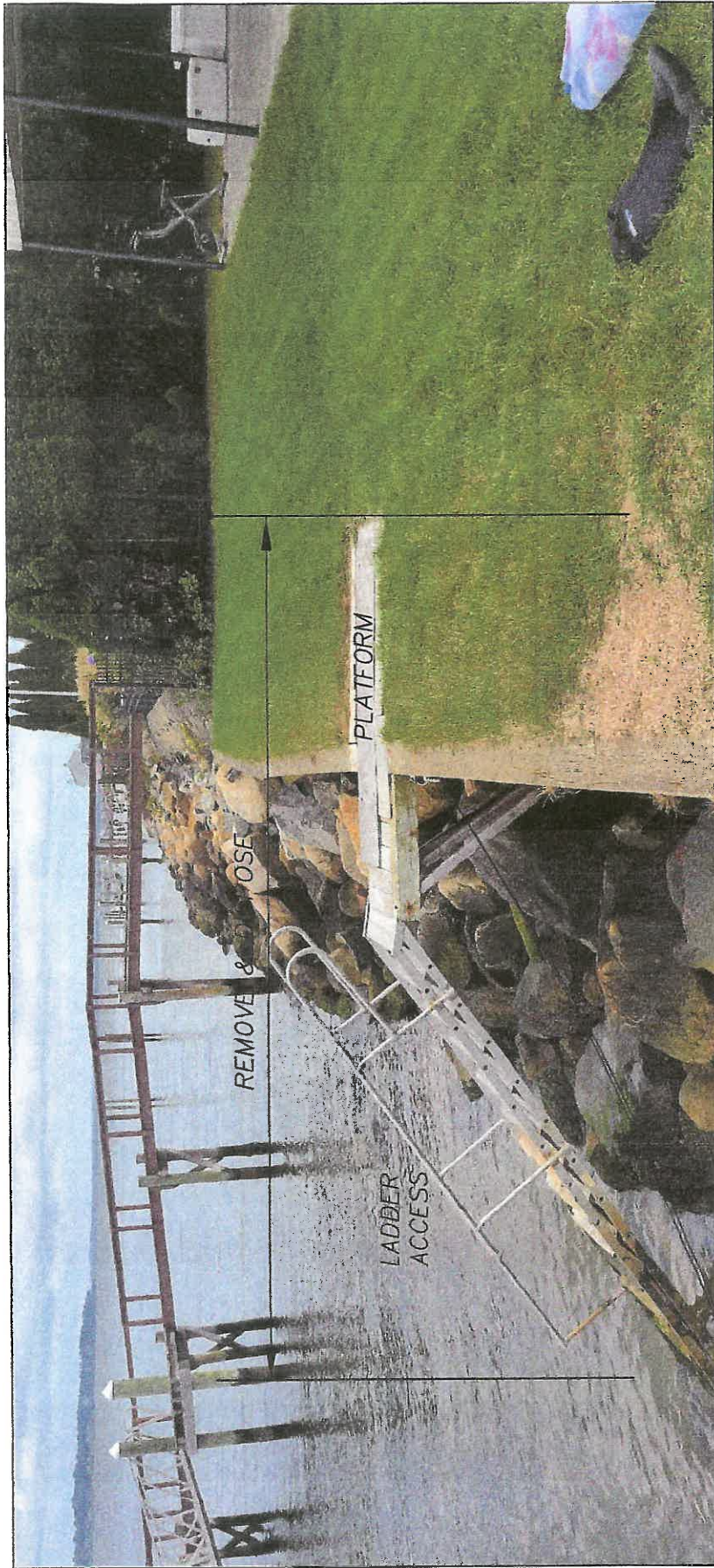
EXISTING 3.5'x8' PLATFORM AND LADDER ACCESS TO BE REMOVED AND DISPOSED
