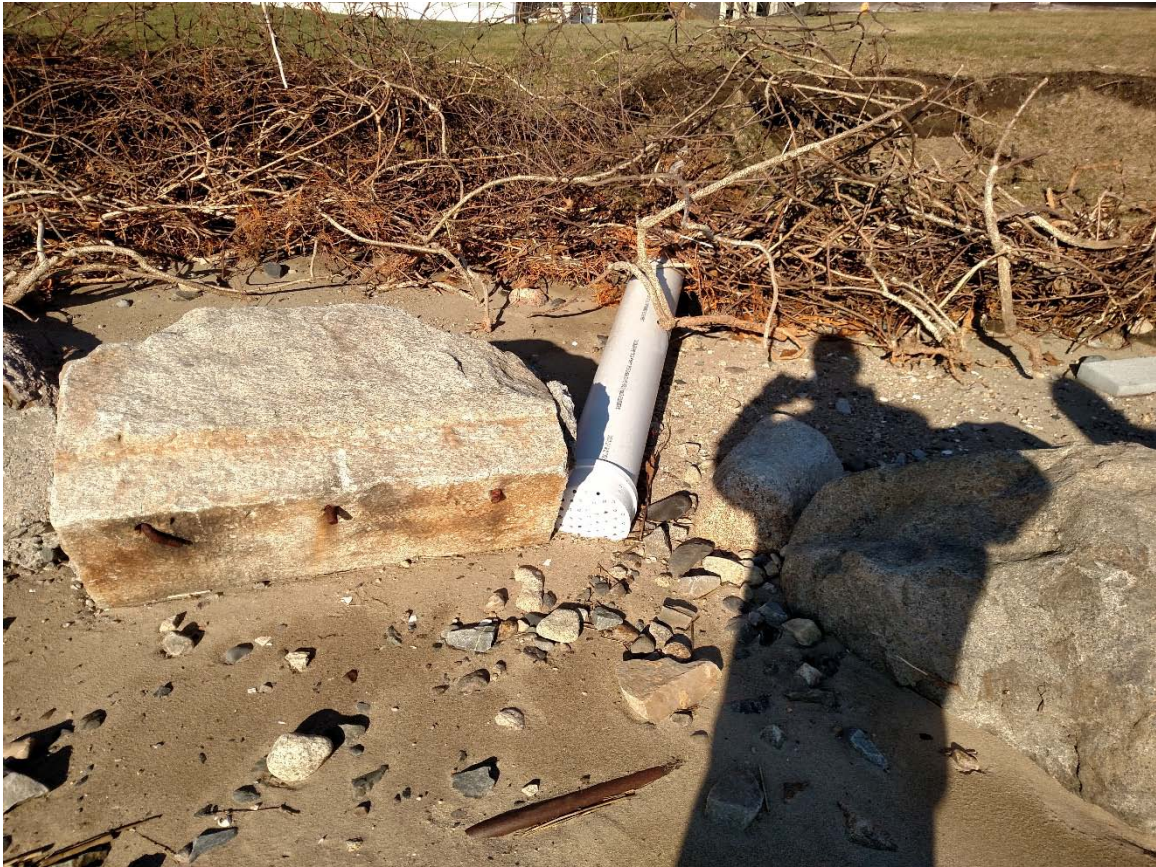
Foundation Pipe Damaged – Was Approx. 2 ft. Above Grade
