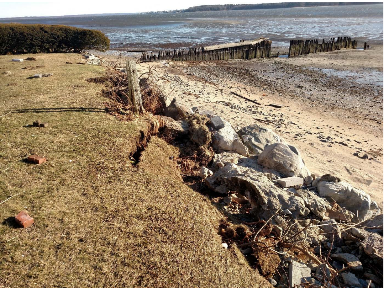
Damage from Monday's Storm 1-17-2022 – Overtopped Stone Revetment – Debris on Lawn
