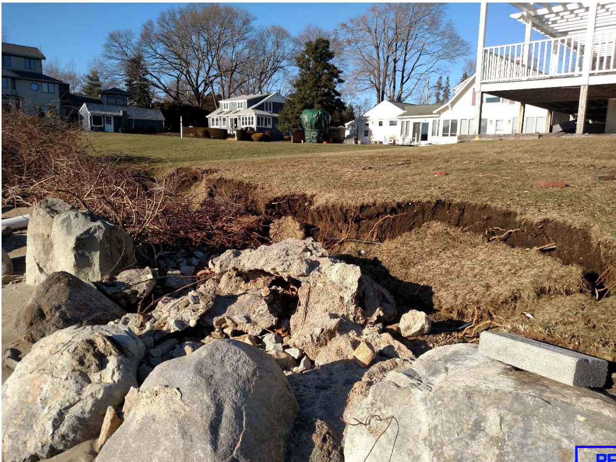
Armor Stones Dislodged and Lawn Damage
