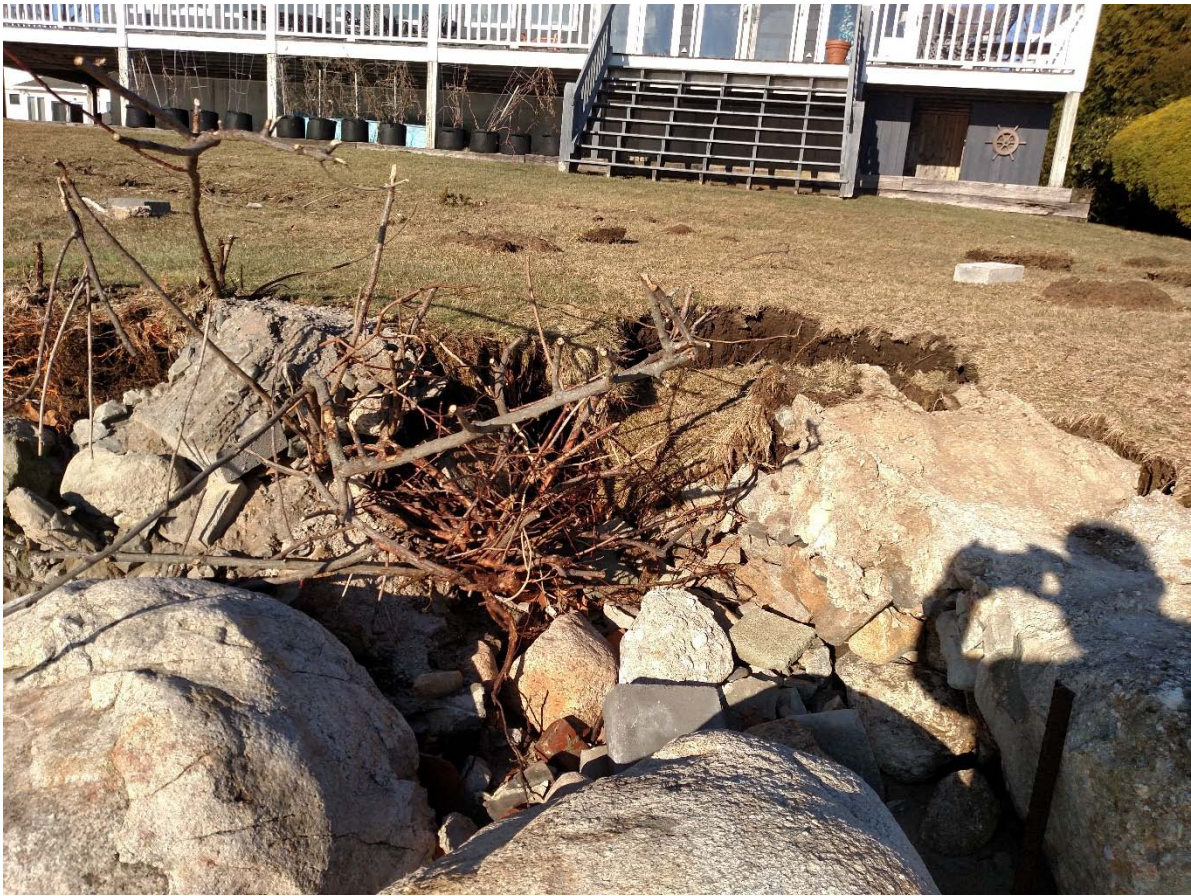
Armor Stones Dislodged and Lawn Damage
