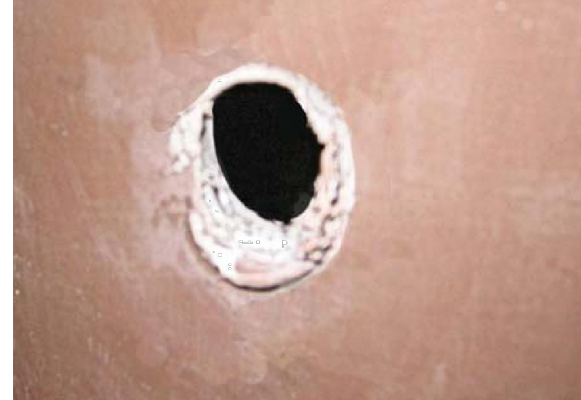
Bolt Hole Elongation - exterior
