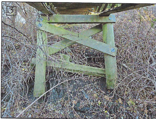
PILE BENT B2 TO BE SISTERED
