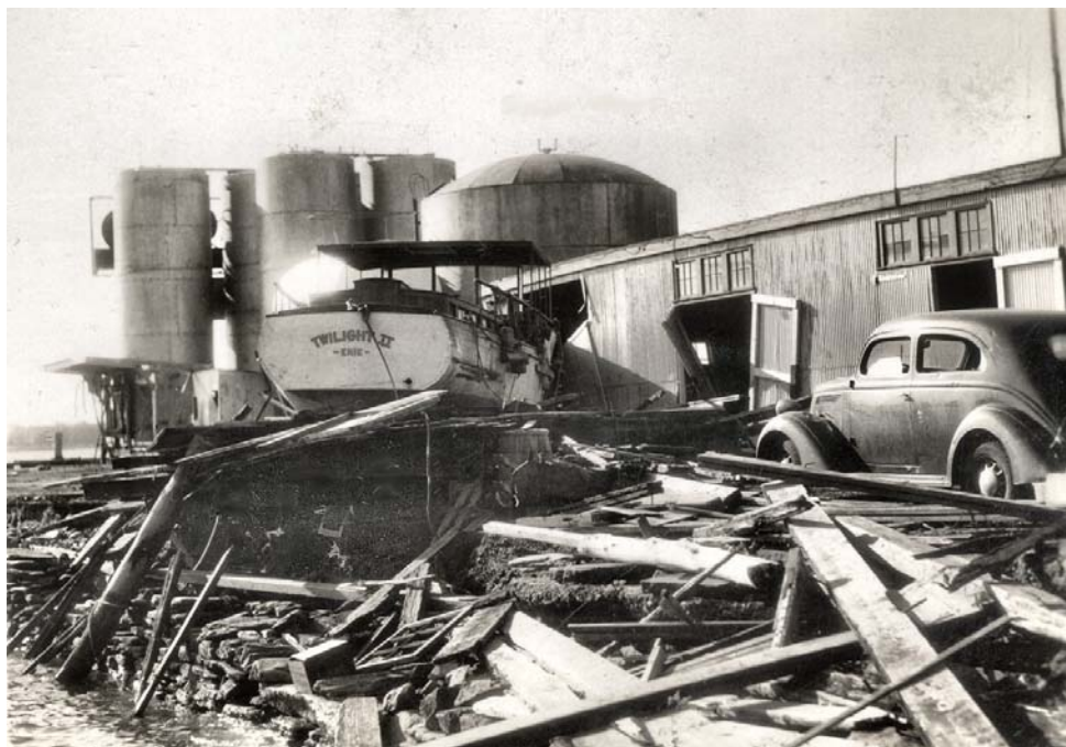
Figure 6. The Great Hurricane of 1938 severely damaged wharves, warehouses and other shoreside facilities throughout the state. (Photo by Providence Journal )
