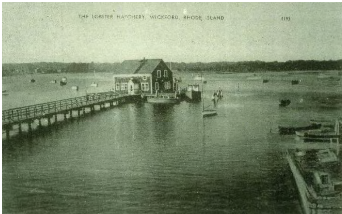
Figure 6. The dock and lobster hatchery building at the end of Fowler Street in Wickford, RI. The historic postcard photo is from the collection of the author.
