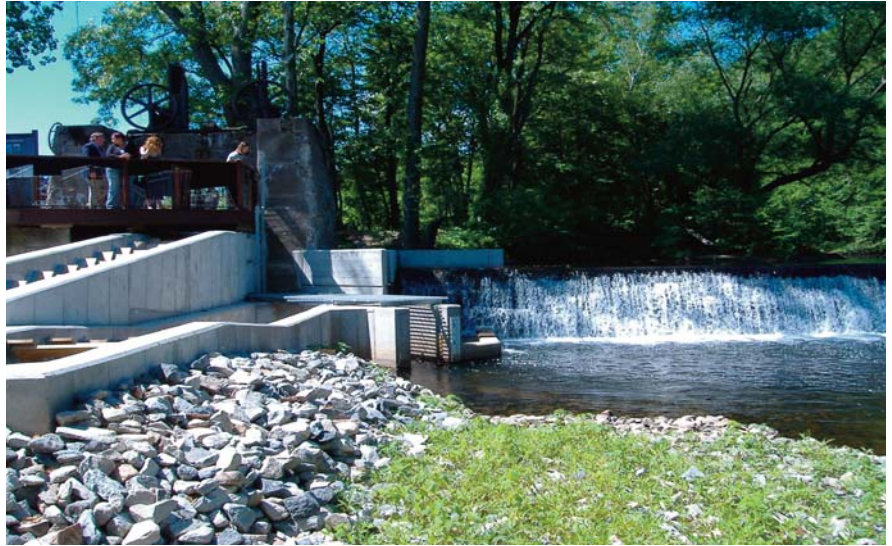
The newly built fish passage at the former Rising Sun Mills in Providence will restore historic anadromous fish runs to the lower Woonasquatucket River.
