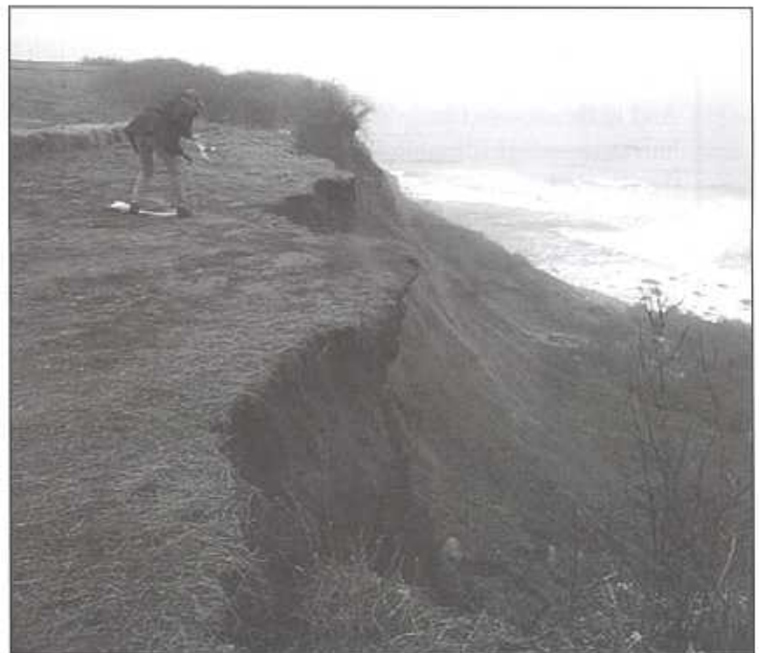
On Edge: Ken Anderson, CRMC Supervising Civil Engineer, takes measurements to establish setbacks from the new edge of the bluff face at the collapse site. Photo: Janet Freedman, CRMC
