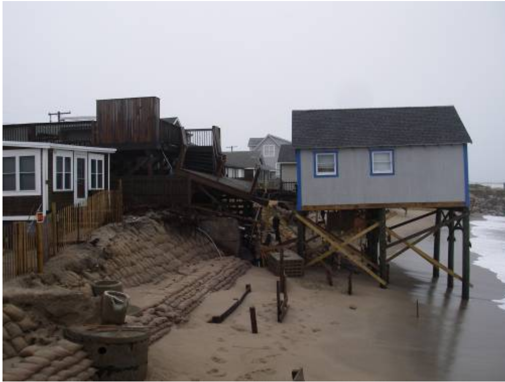
Figure 19. The same structures in 2010 as shown in Figure 18 above. Approximately twenty feet of bluff landward of the house has eroded since 1999.
