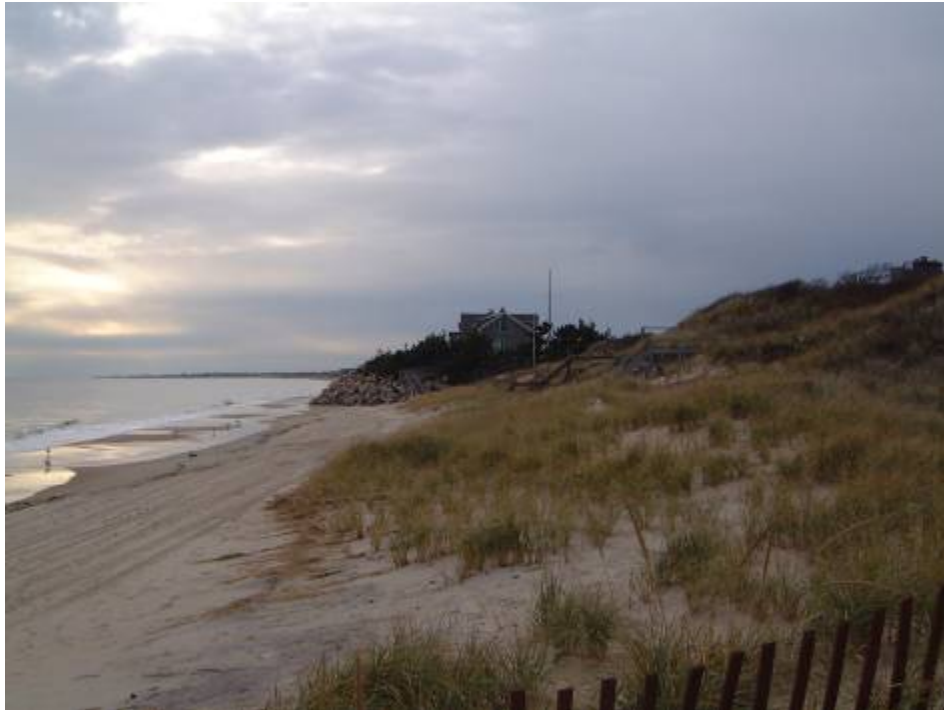
Figure 1. Lateral access obstruction in front of a shoreline protection structure in Westerly
