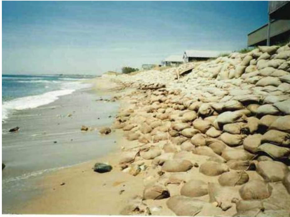
Figure 15. Emergency erosion control west of Deep Hole after 1999 extra-tropical storm.
