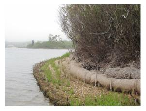
Bioengineering or soft engineering techniques include the use of biodegradable materials such as jute and coir fibers to protect shorelines from erosion. Coir logs are made from woven coconut fiber and can be used at the base of an eroding bank or salt marsh. This is an example of a project in Charlestown, RI where a combination of coir logs and marsh grass was used.
