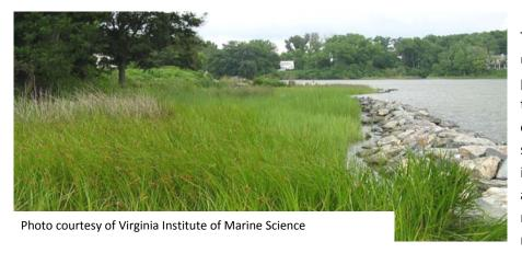
The marsh sill technique utilizes stone as erosion protection at the edge of the marsh. The design is often segmented or offset so that habitat continuity is not interrupted and fish and other animals can move in and out of the marsh. The example
