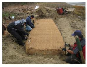
Coir envelopes are coir fabric filled in place with locally compatible sand and then stitched together, holding the sand in place. These envelopes can then be used to create a terraced bank where natural material and sand absorb wave energy and reduce erosive wave reflection. Coir envelopes should be planted or seeded with native grasses or coastal shrubs to prevent breakdown of the material by UV exposure. This is an example from Byway Road in Barrington, RI.
