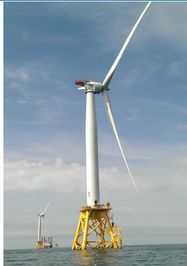
A view of the Block Island Wind Farm
