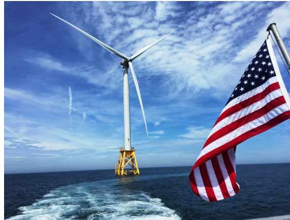
Block Island Wind Farm turbine 1
