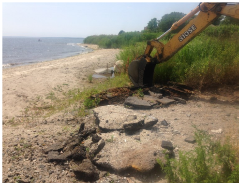
Van Zandt Avenue, Warwick, where eroded pavement was removed and a filter strip was installed in 2017. (Photo: CRMC, Save The Bay)
