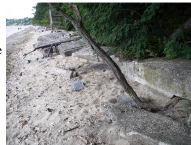
A section of an older, failed revetment
