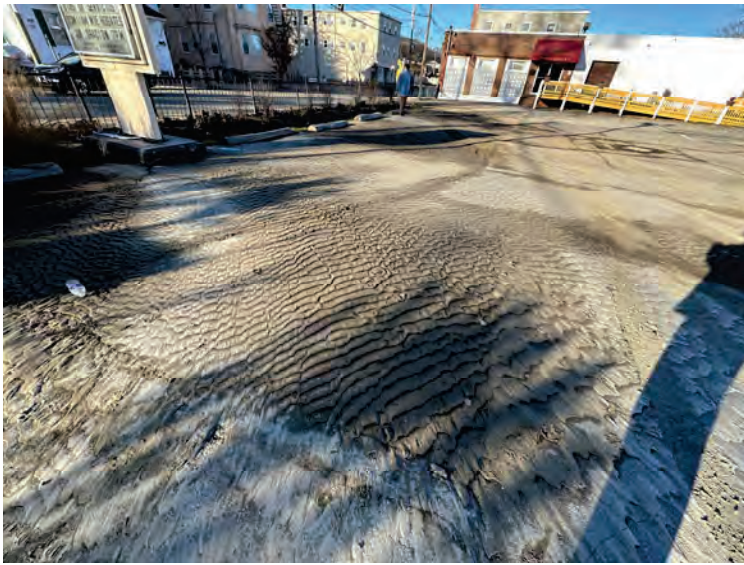
FIGURE 1K - RECENT FLOOD EVENTS LEFT SIGNIFICANT AMOUNTS OF SILT, SAND AND OTHER SEDIMENT IN UPLAND AREAS, WHICH INCLUDED STORMWATER MEASURES INSTALLED BY WRWC IN 2020 NEAR DONIGIAN PARK.
