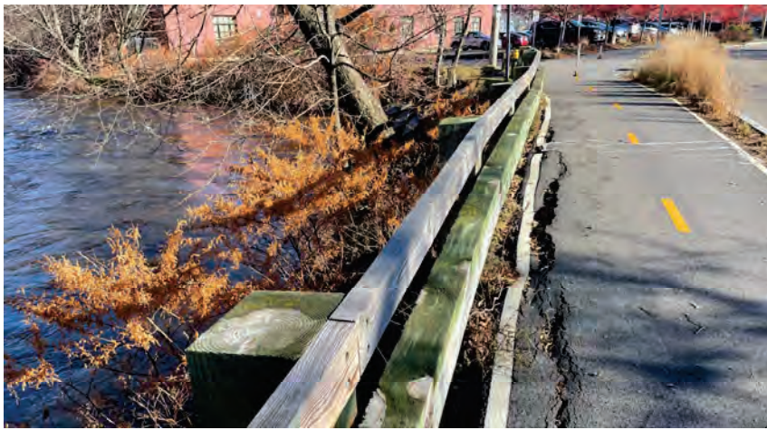
FIGURE 1A – SEPARATED BIKE PATH (WOONASQUATUCKET RIVER GREENWAY SPUR) ALONG SAN SOUCI DRIVE. SINKING AND CRACKING OF PAVEMENT AS A RESULT OF BANK EROSION VISIBLE. PHOTO TAKEN AFTER DECEMBER 18, 2023 RAINFALL EVENT.
