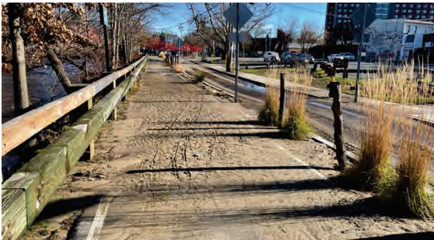
FIGURE 1D – VIEW LOOKING EAST ALONG SAN SOUCI DRIVE AFTER THE DECEMBER 18, 2023 RAINFALL EVENT. SEDIMENT ON BIKE PATH AND ROAD SHOW THE EXTENT OF FLOODING.
