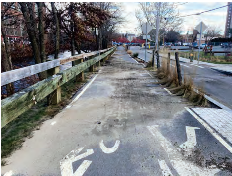
FIGURE 1J – – VIEW LOOKING EAST ALONG SAN SOUCI DRIVE AFTER THE JANUARY 10, 2023 RAINFALL EVENT. SEDIMENT ON BIKE PATH AND ROAD SHOW THE EXTENT OF FLOODING.
