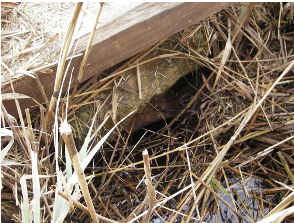
Figure C18: Site 1165- culvert leading into Site 1161 across the road.
