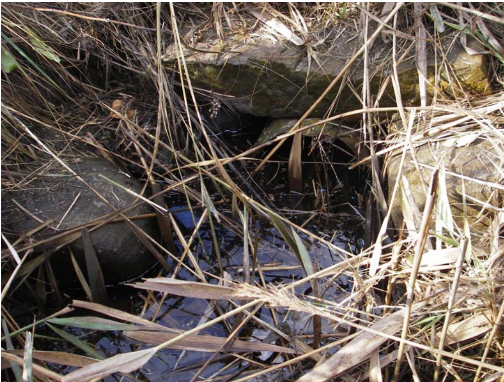
Figure C16: Site 1161- view of the culvert allowing flow into and out of the site.
