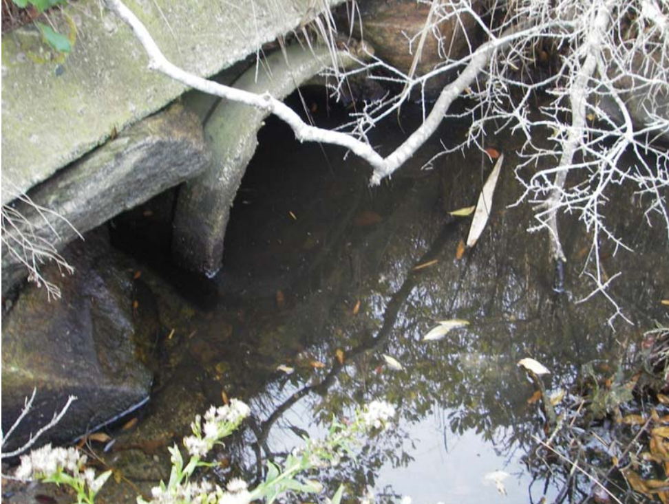
Figure C9: View of Site 696 across the street from Site 682, showing a culvert that leads into the wetland area.
