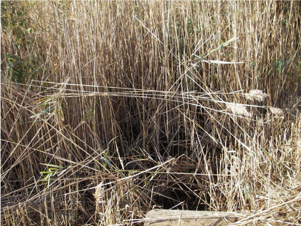
Figure C17: Site 1161- edge of culvert box with ponded water and most of the site being covered by Phragmites .
