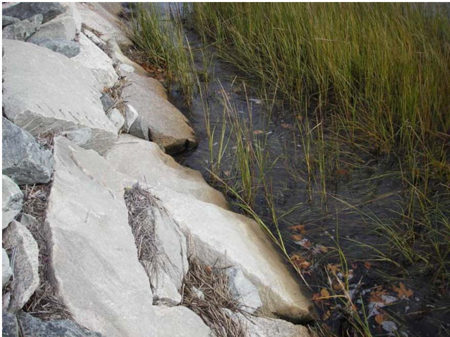
Figure C2: Across the street from Site 158, there is no obvious culvert but water is seeping under the road.
