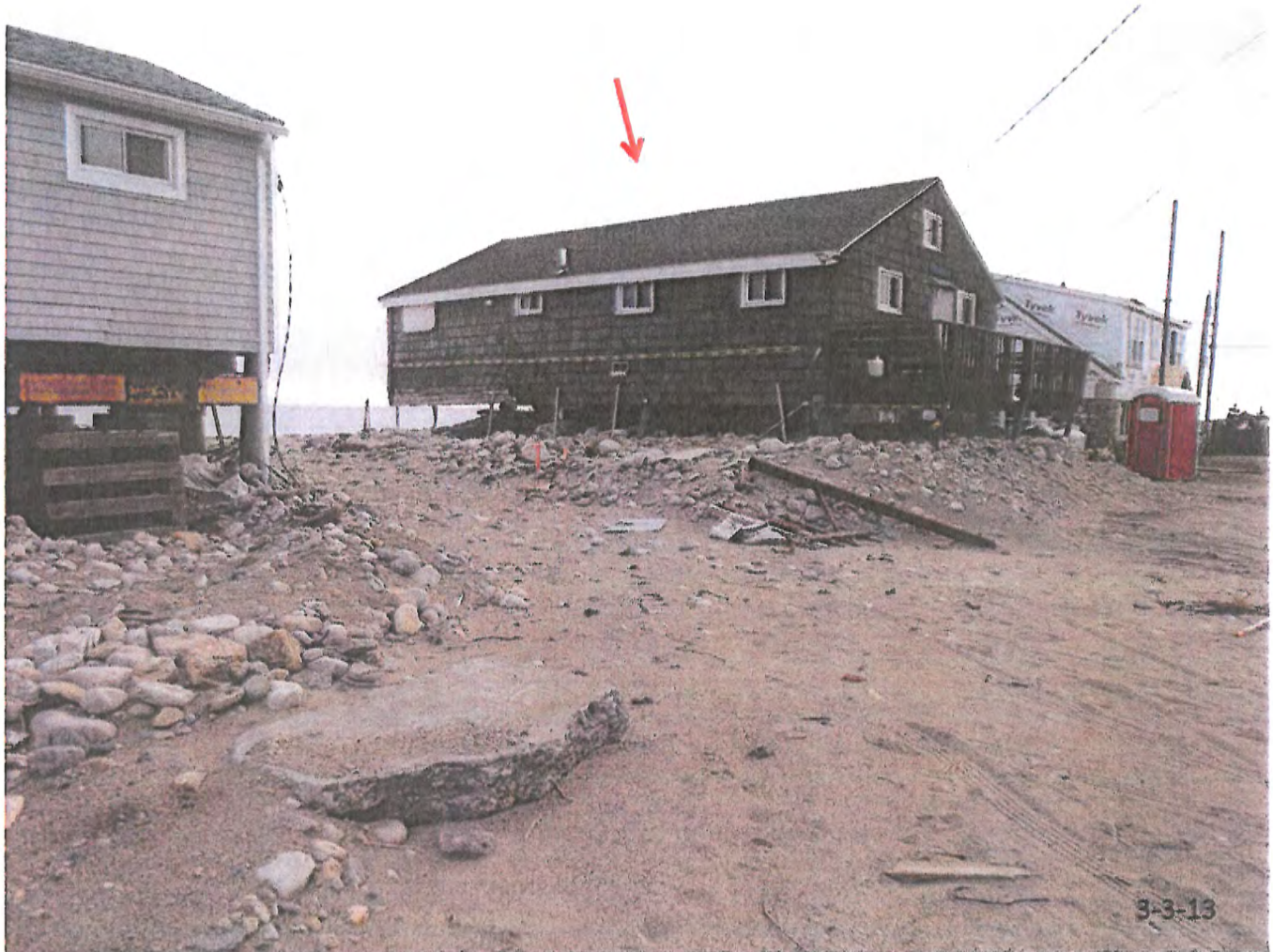
Figure 10. The applicant's property prior to demolition several months after Sandy.
