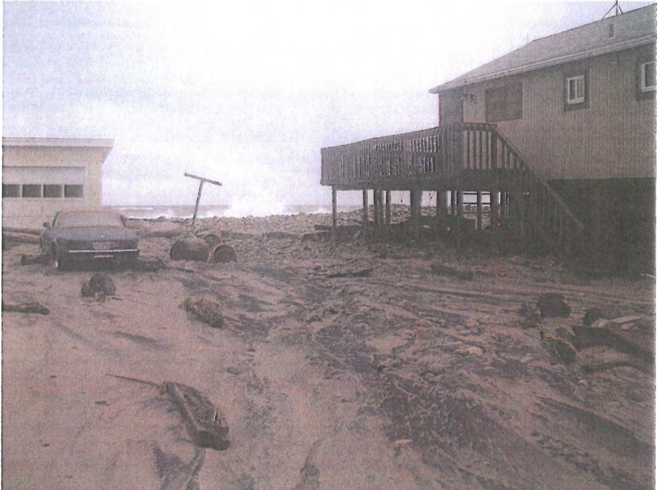
Figure 6. Overwash sand is eroded from the beach and dune by storm surge and waves is deposited landward of the houses during the Patriot Day Nor'easter in 2007. The house on the right is next door to the applicant's property.
