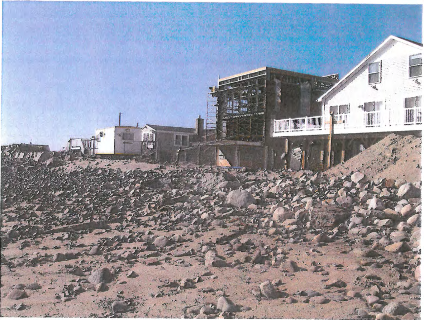
Figure 11. The applicant's property (c/m Assent 2016-09-116) after a nor'easter in October 2017.
