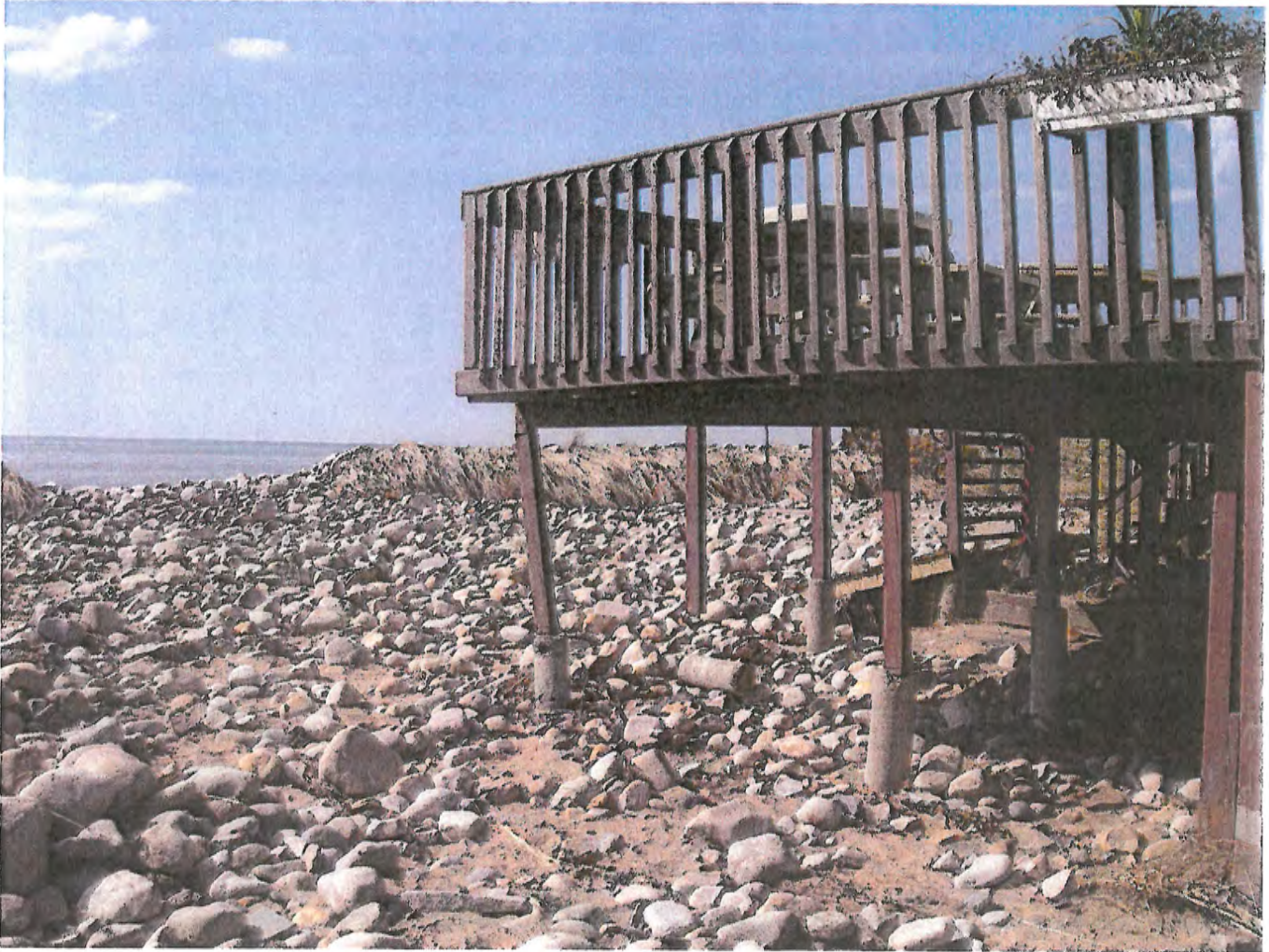
Figure 7. Sand and cobble from the beach and dune was eroded during Tropical Storm Irene in 2011. The post-Irene beach was characterized by cobble and boulder. Remnants of the dune remained at the next door property, but the exposed base of the pilings indicate that there was erosion in the back dune area as well as on the beach.
