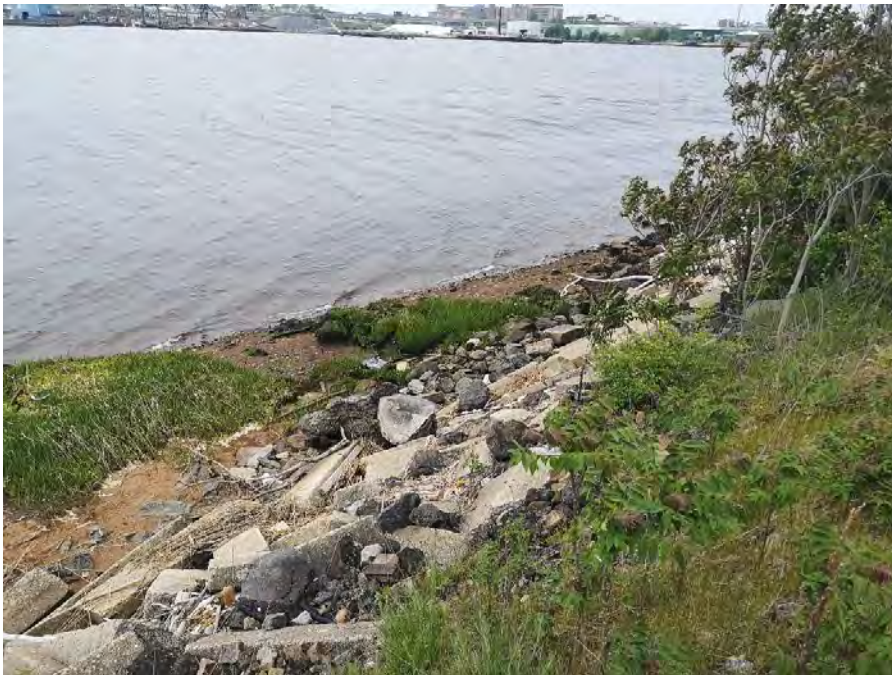
Photo No. 10 – Northwestern embankment looking west
