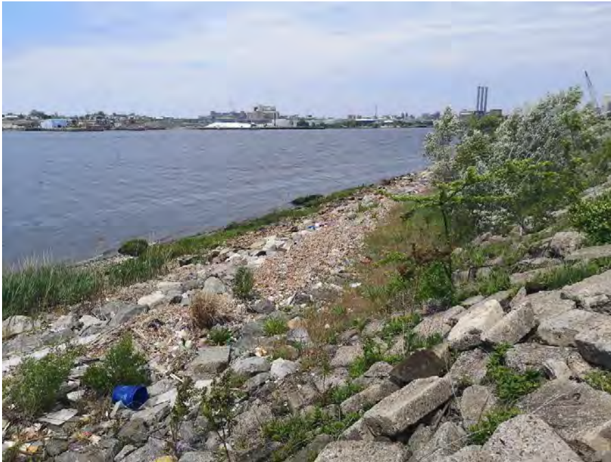
Photo No. 7 – Southwestern Embankment Looking north
