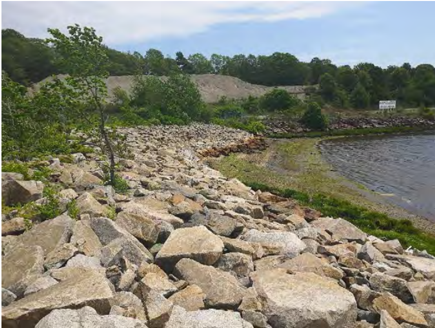
Photo No. 1 – Southern Embankment looking east
