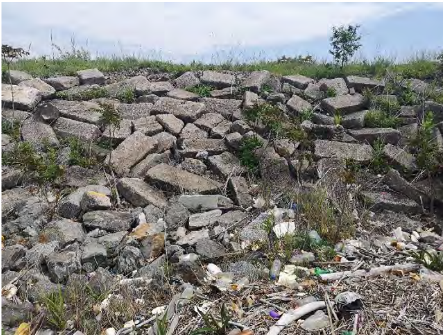
Photo No. 8 – Southwestern Embankment Looking East
