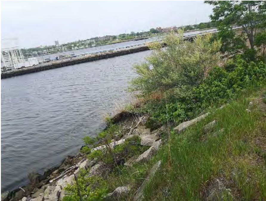
Photo No. 11- Northwestern embankment looking north
