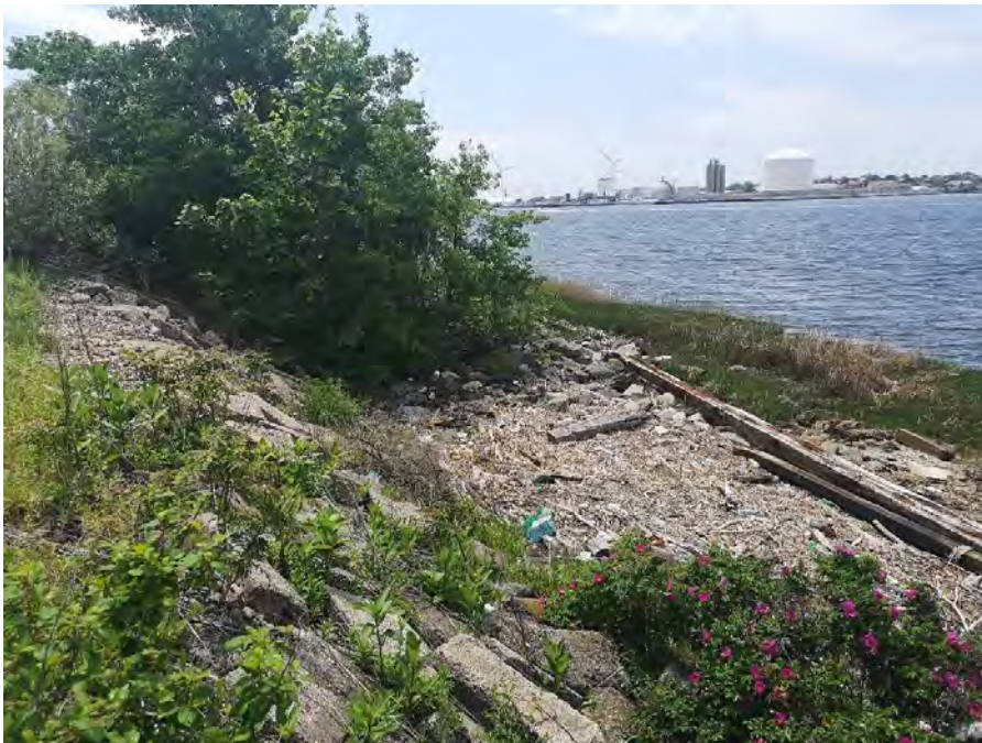
Photo No. 6- Southwestern part of embankment looking south
