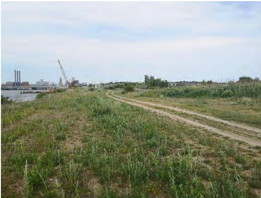
Photo No. 12 – Top of embankment looking north
