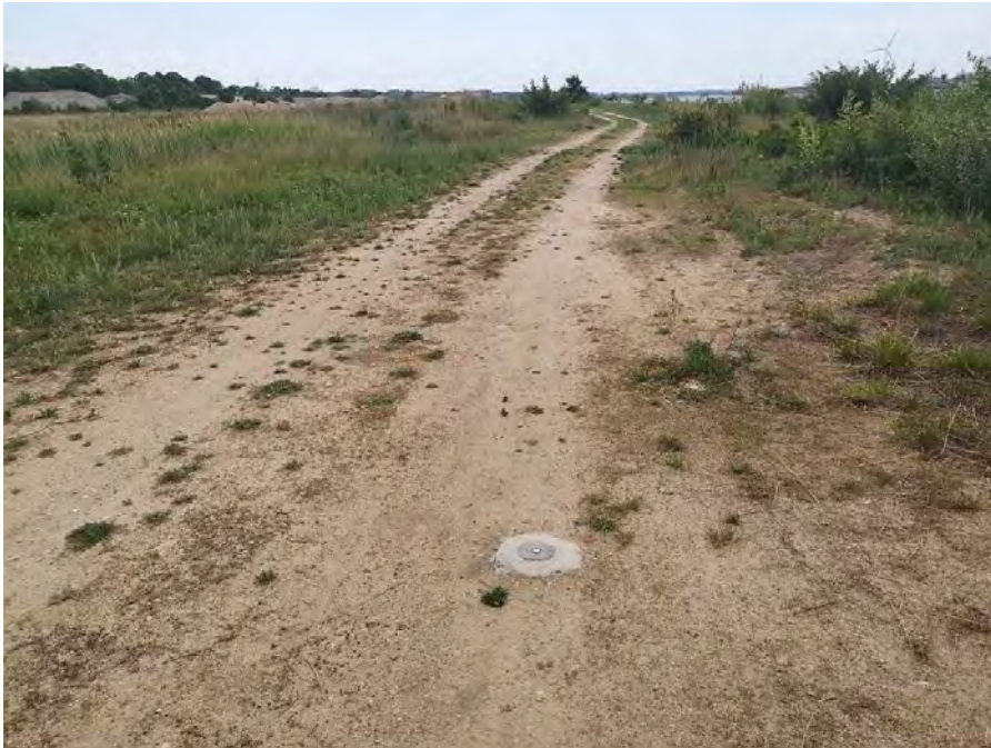
Photo No. 13 – Top of embankment looking south
