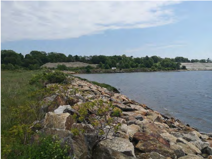
Photo No. 3 – Southern Embankment looking east
