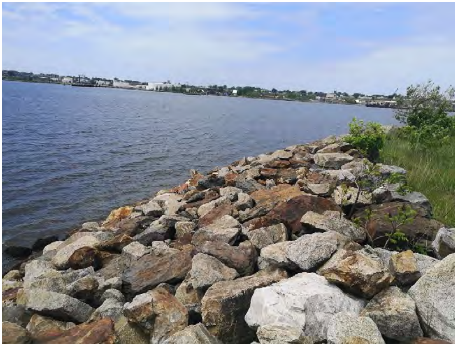
Photo No. 4- Southern Embankment Looking West
