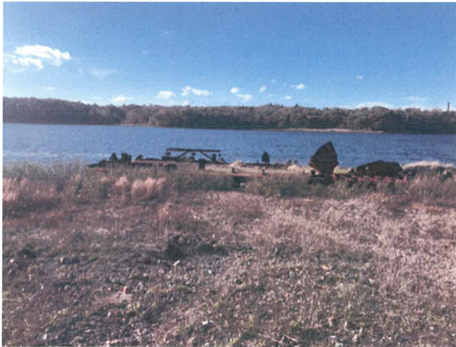
Photo 4: View west of barge to be removed
