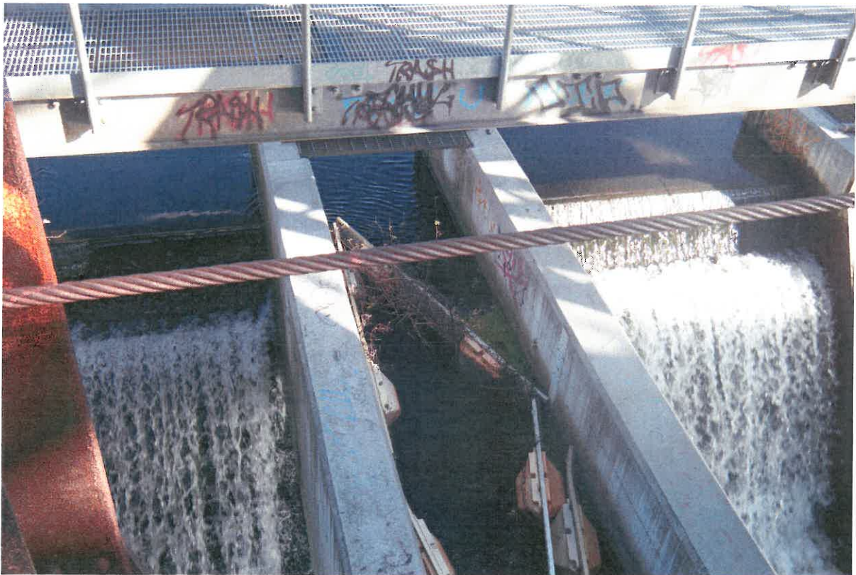
Photo 10: Omega Pond dam
