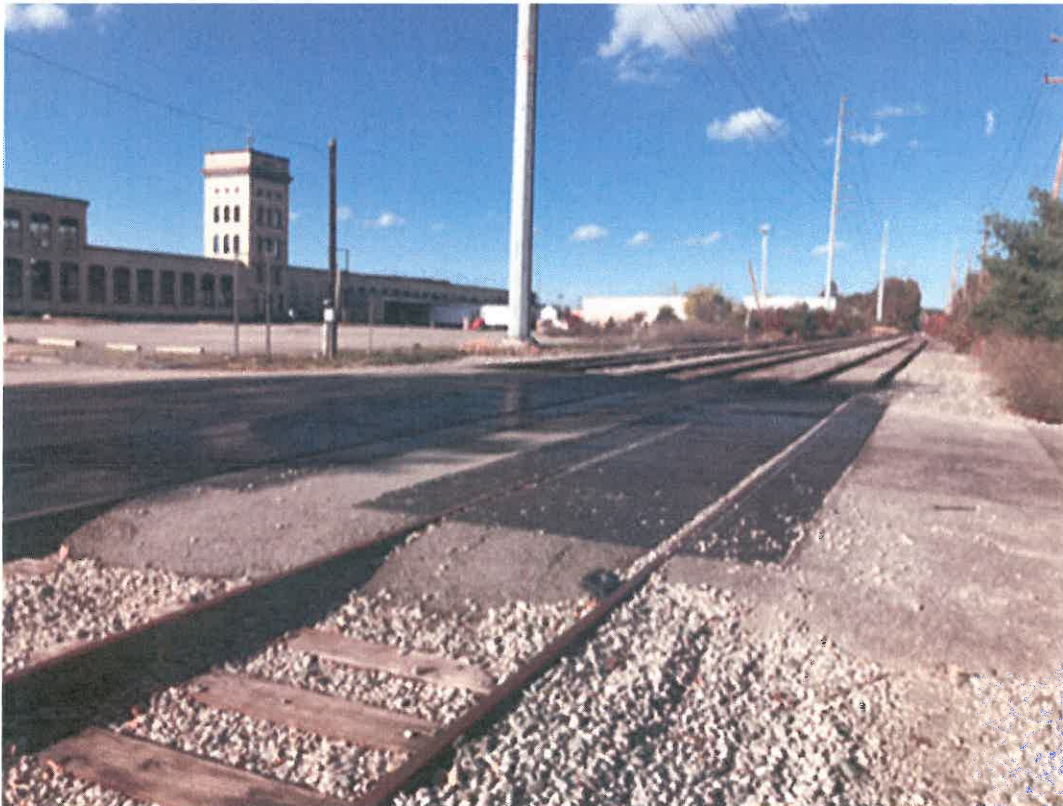
Photo 8: View north from RR track crossing
