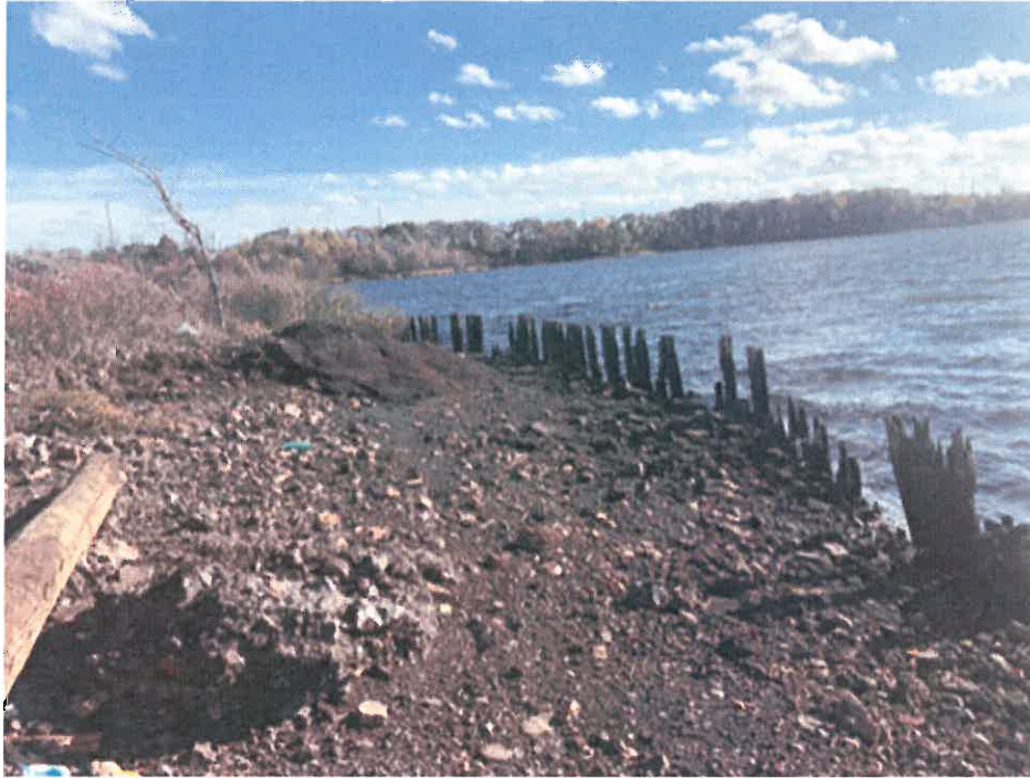
Photo 5: View east along Coastal Side timber bulkhead
