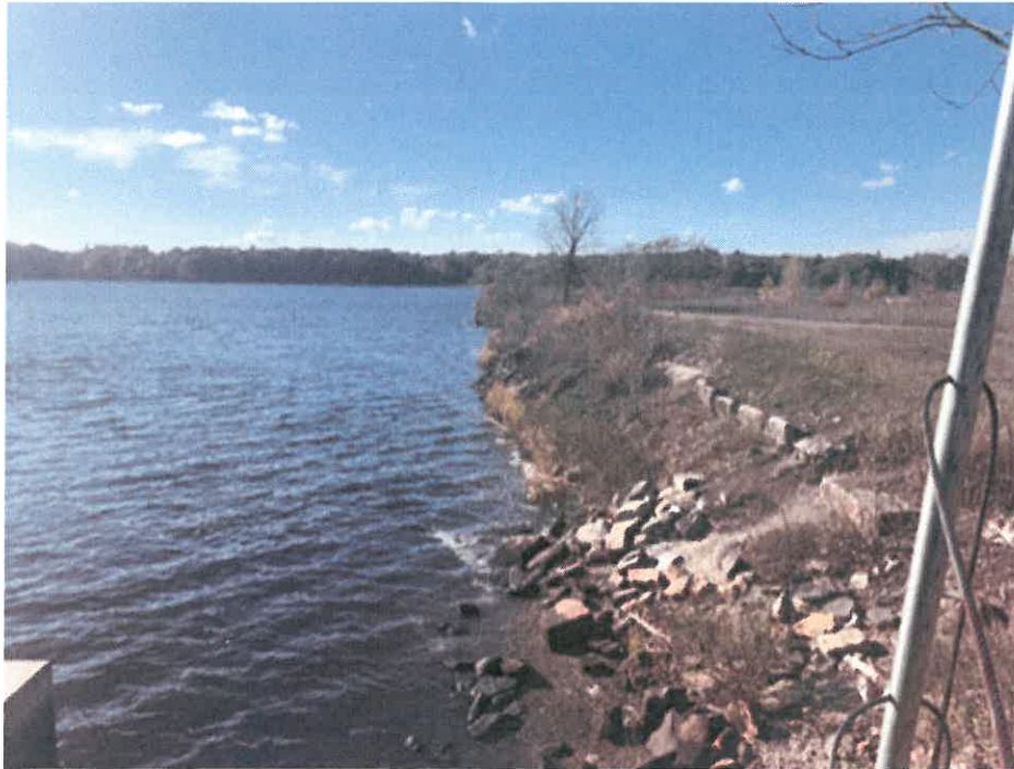
Photo 1: View from southeast end of Coastal Side looking west
