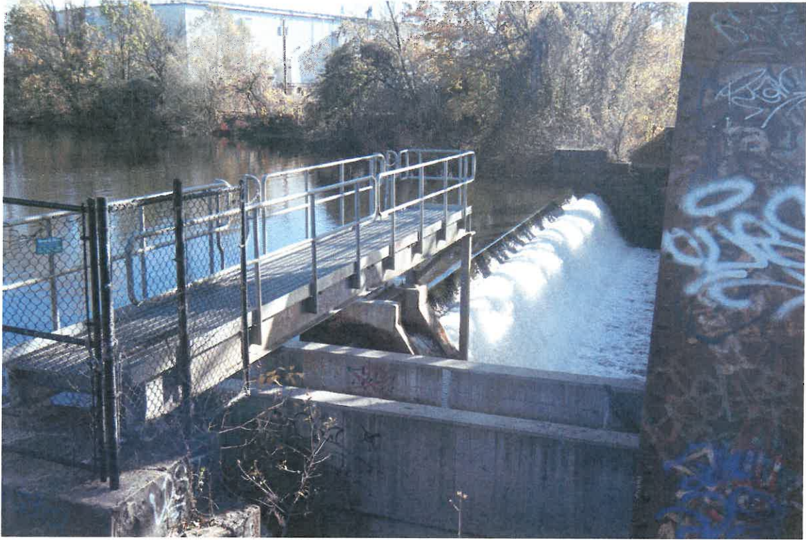
Photo 9: Omega Pond Dam
