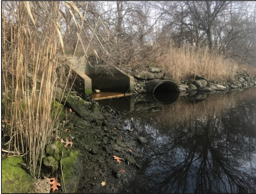
Photo 9: Stormwater outfalls at southwest of North Landfill (near WF # CF 9)
