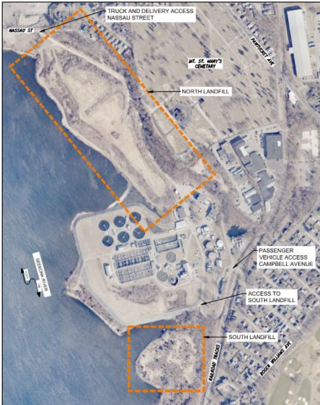
Figure 1-2 Bucklin Point North and South Landfills
