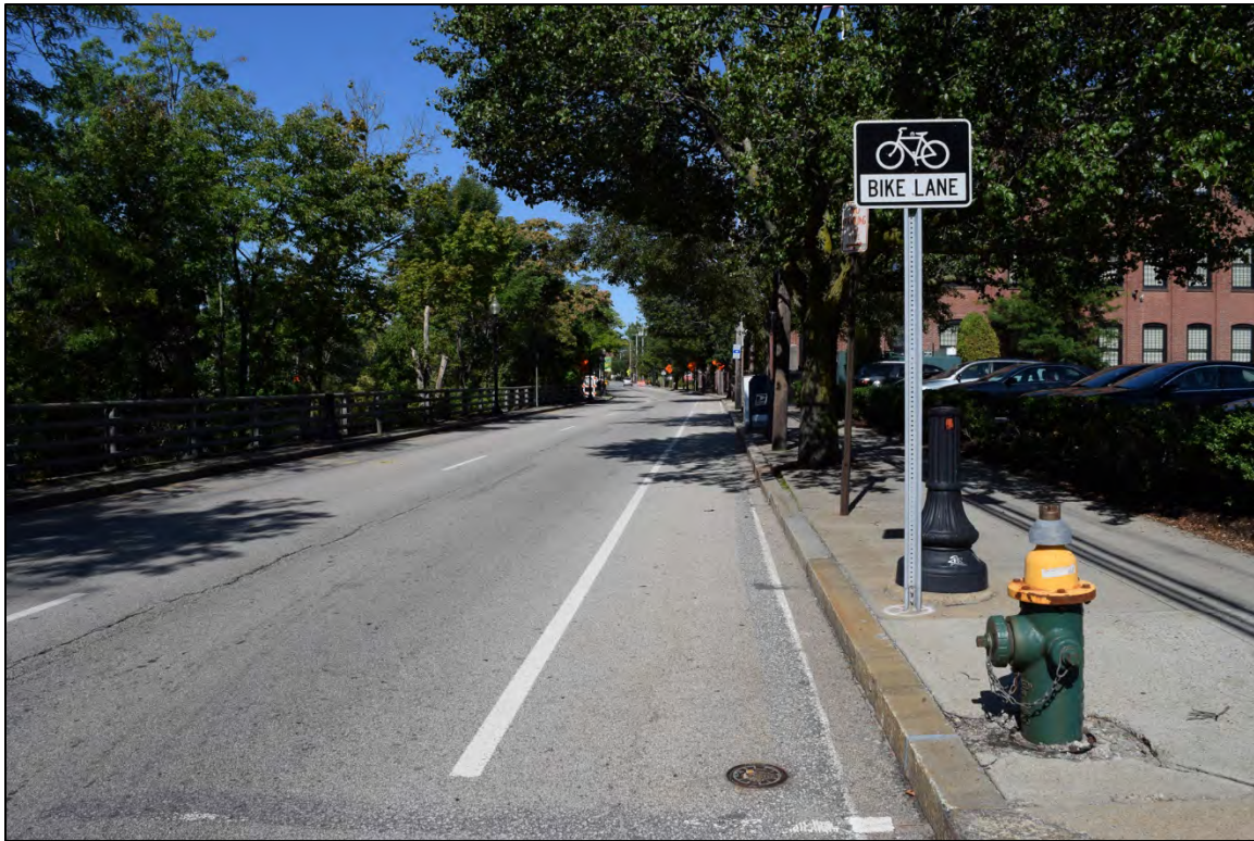
Photo 1. Woonasquatucket River Greenway on Promenade Street, view west.
