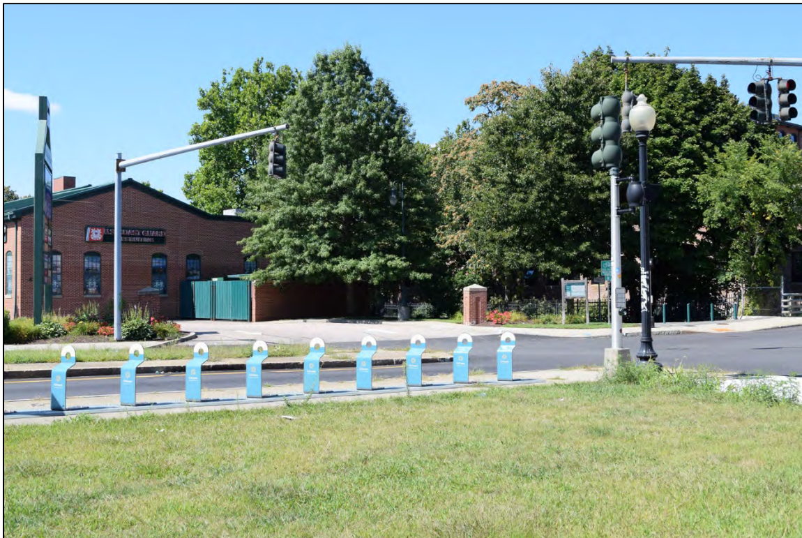
Photo 16. View of the Valley Worsted Mill (Part of Eagle Square Buildings) (Map No. 6) with the Woonasquatucket River Greenway immediately north, view northwest.
