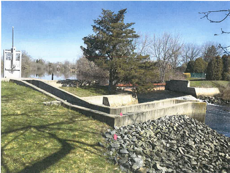
Photo 6: View of the fishway structure and dam facing north.
