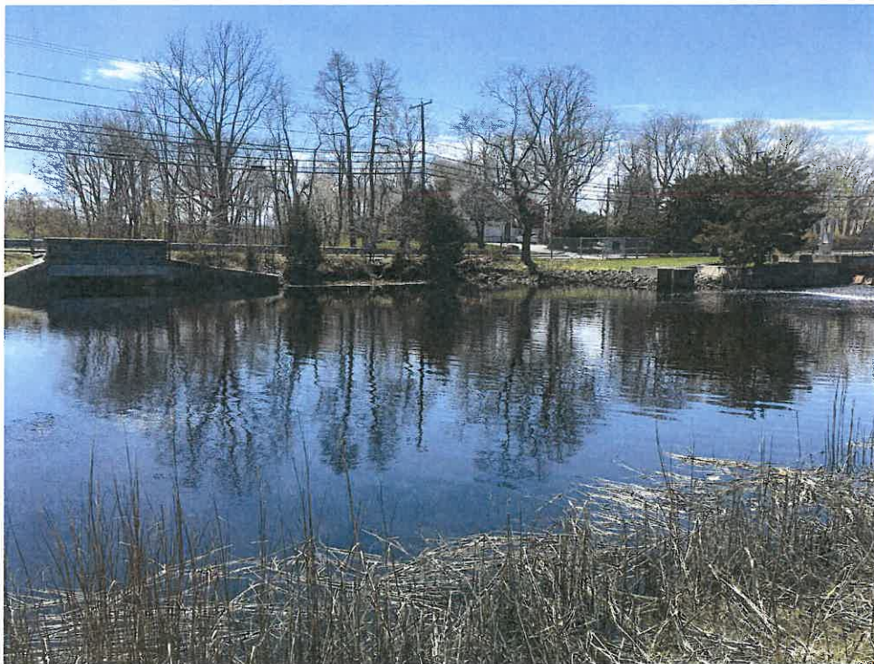
Photo 2: View of the tidal Kickemuit River and Child Street culvert facing southwest.
