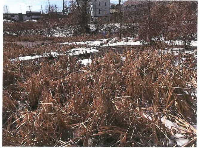
Photo 31. Southwesterly view across upper and western portions of the Basin, showing breadth of heavy sediment accumulation. The project proposes to remove the accumulated sediment down to the concrete liner and to restore the Basin side slopes to original grades.
