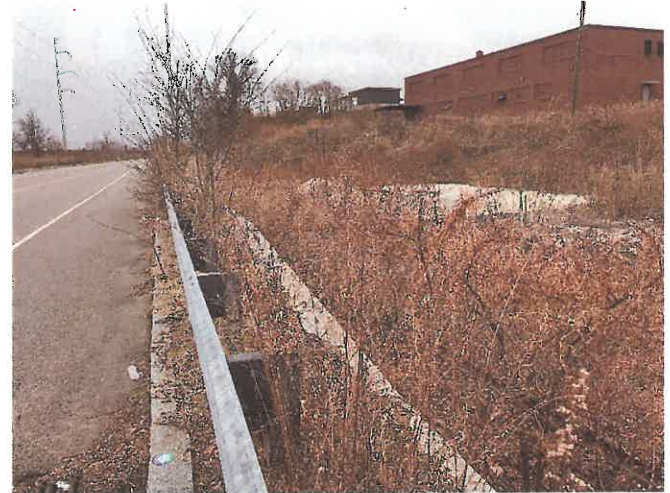
Photo 44. Northerly view along Waterfront Drive showing general setting, concrete retaining wall, and elevation difference noted in Photo 43.
