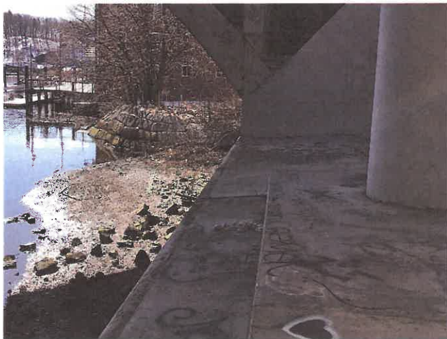
Photo 12. Southerly view showing a close-up of the EB pier foundation and significant elevation drop to the intertidal substrates shown in Photo 10.
