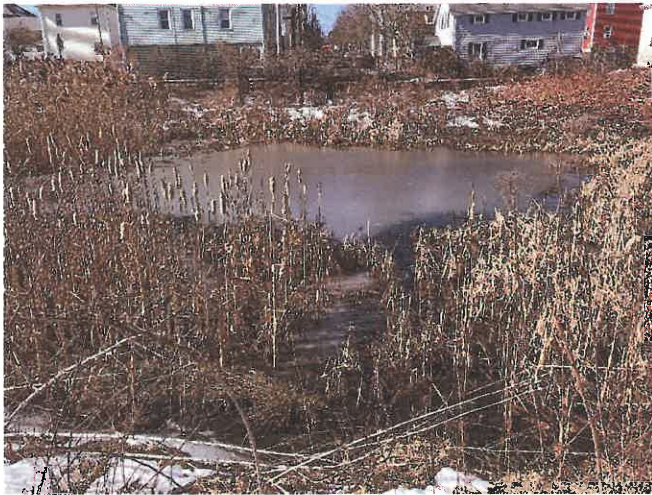
Photo 32. Westerly view across the Storage Pond, the middle compartment of the water quality ponds. No work is proposed in this compartment.
