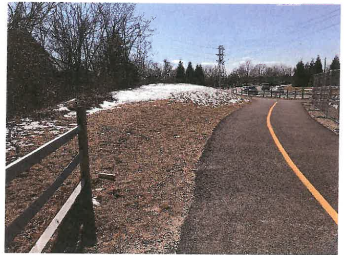
Photo 36. Opposite (southerly) view of that shown in Photo 35. The elevated topography to the left will help ensure that secondary effects, such as errant stormwater runoff, do not impact the Boathouse property to the east (left). The end of the split rail fence is helpful for reference with Photo 35.
