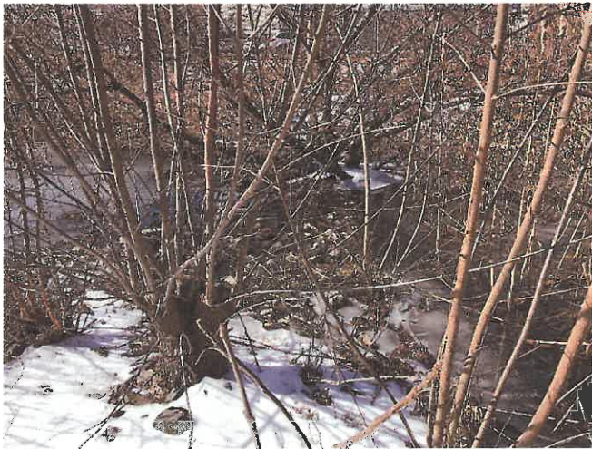
Photo 34. Westerly view of the stone weir positioned between the Storage Pond and Micropool. The weir is proposed to be reshaped to original design specifications.
