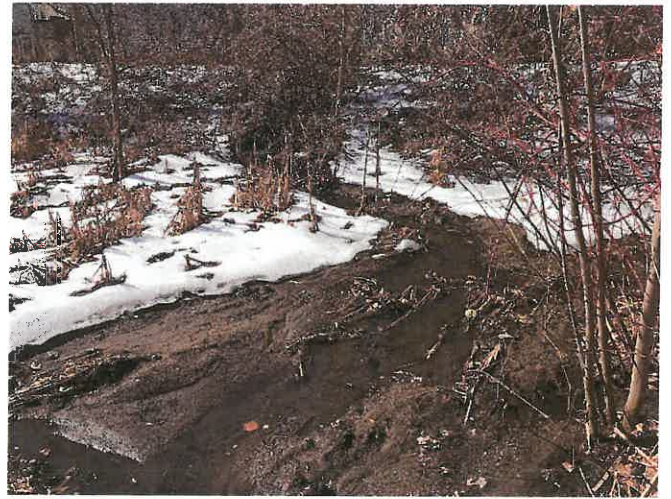
Photo 29. Northwesterly view of northern inlet, with flow restricted by heavy sediment deposits.
