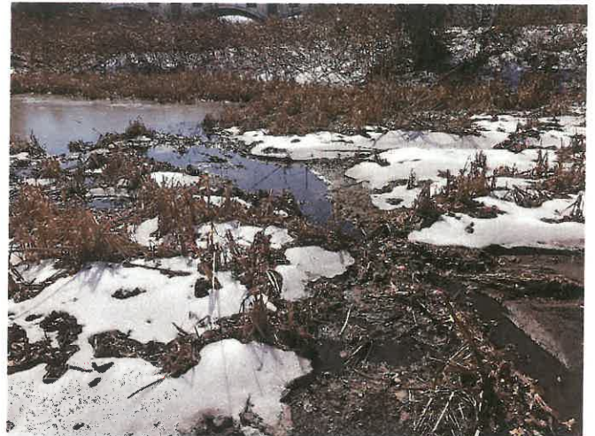
Photo 27. Southerly view of severe sediment accumulation. Flow from the northern inlet is shown at lower right, and the mouth of flow from the western inlet is somewhat discernable two-thirds up image at right.
