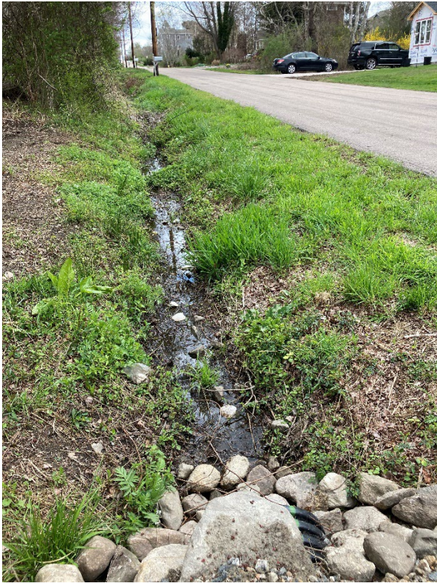
4. Photo of site looking southeast taken April 27, 2022 by Devon Robinson
