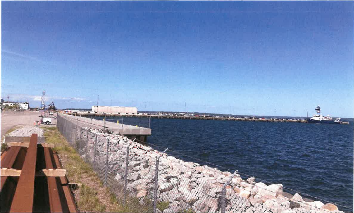
View of proposed Pier location from Terminal 5 (Looking Northeast)
