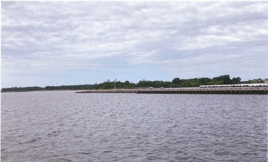
View of Terminal 5 from Pier 1 (Looking Southwest)
