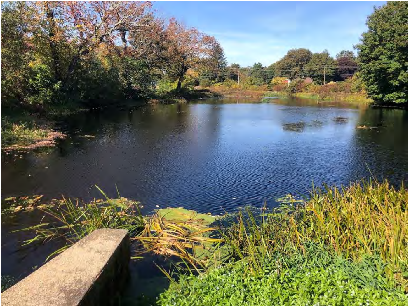
Figure 4: View northwest of the impoundment looking upstream from dam structure. Photo taken November 8, 2022.
