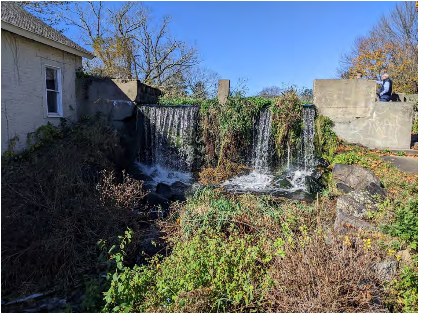
Figure 3: Photo taken during November 8, 2022 site meeting of the Rodman Mill Dam spillway, within the Annaquatucket River in North Kingstown. Property owner Michael Baker is located in the top right corner of the photograph describing site conditions.
