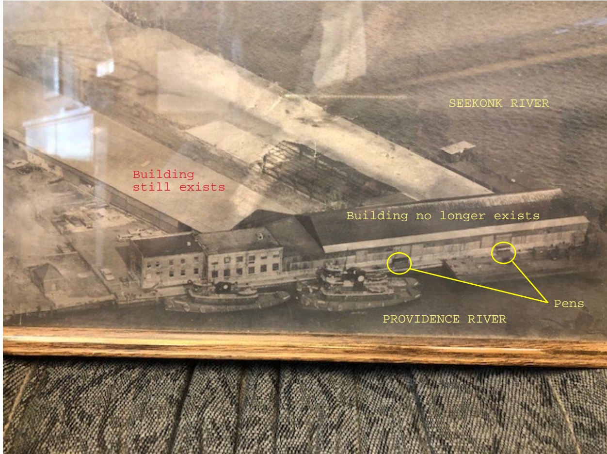
Photo 10: Aerial photograph from 1955 showing port area conditions when the building along the waterfront was still in place. Note the concrete pen areas at the face of the building.
