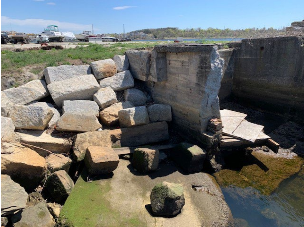
Photo 4: Stone revetment just north of the north concrete pen.
