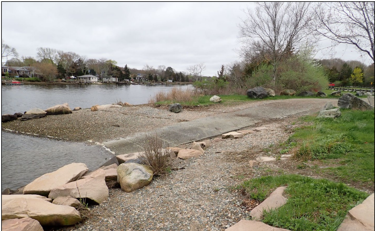
Photo 2: The concrete boat ramp looking southeast.
