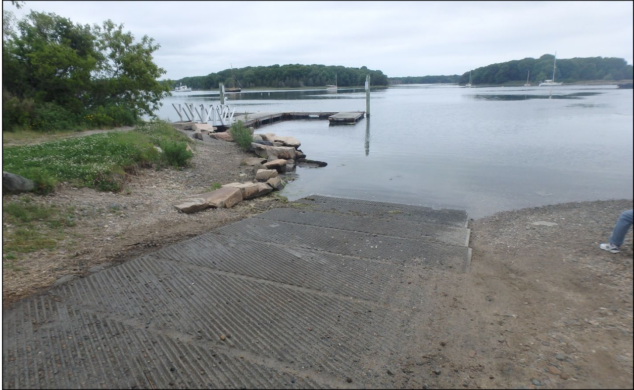
Photo 5: The floating docks as seen from the concrete boat ramp.
