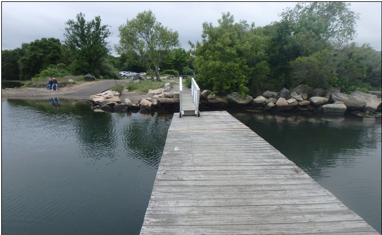
Photo 6: Stone revetment in front of floating dock gangway.
