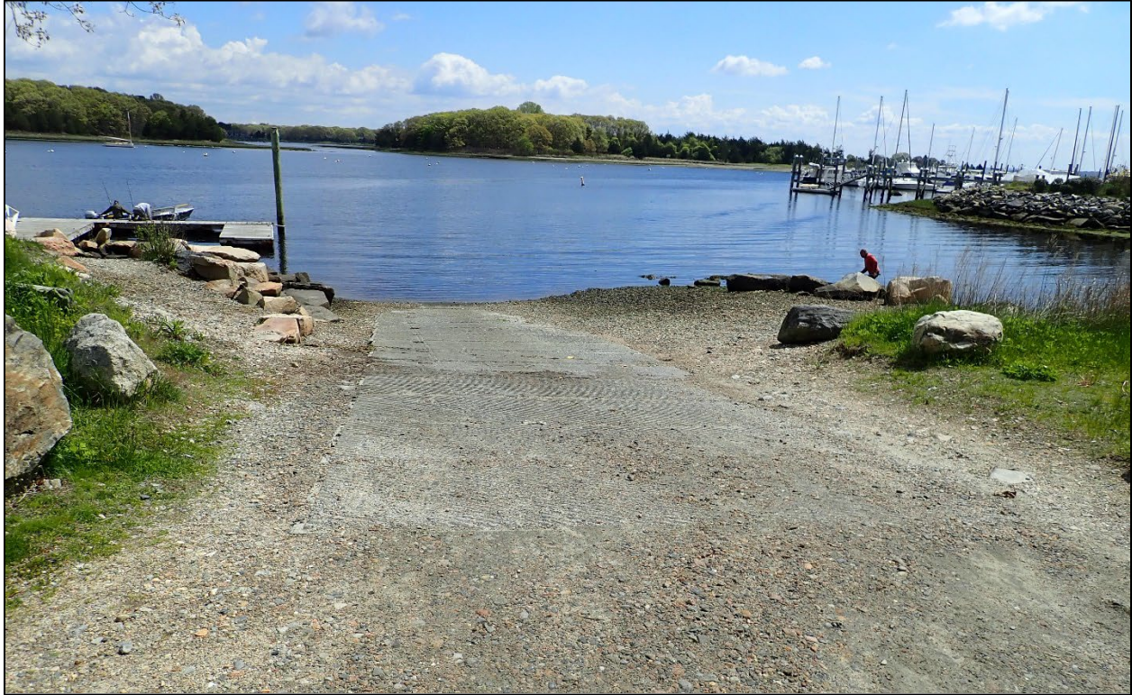
Photo 1: The concrete boat ramp looking northeast.
