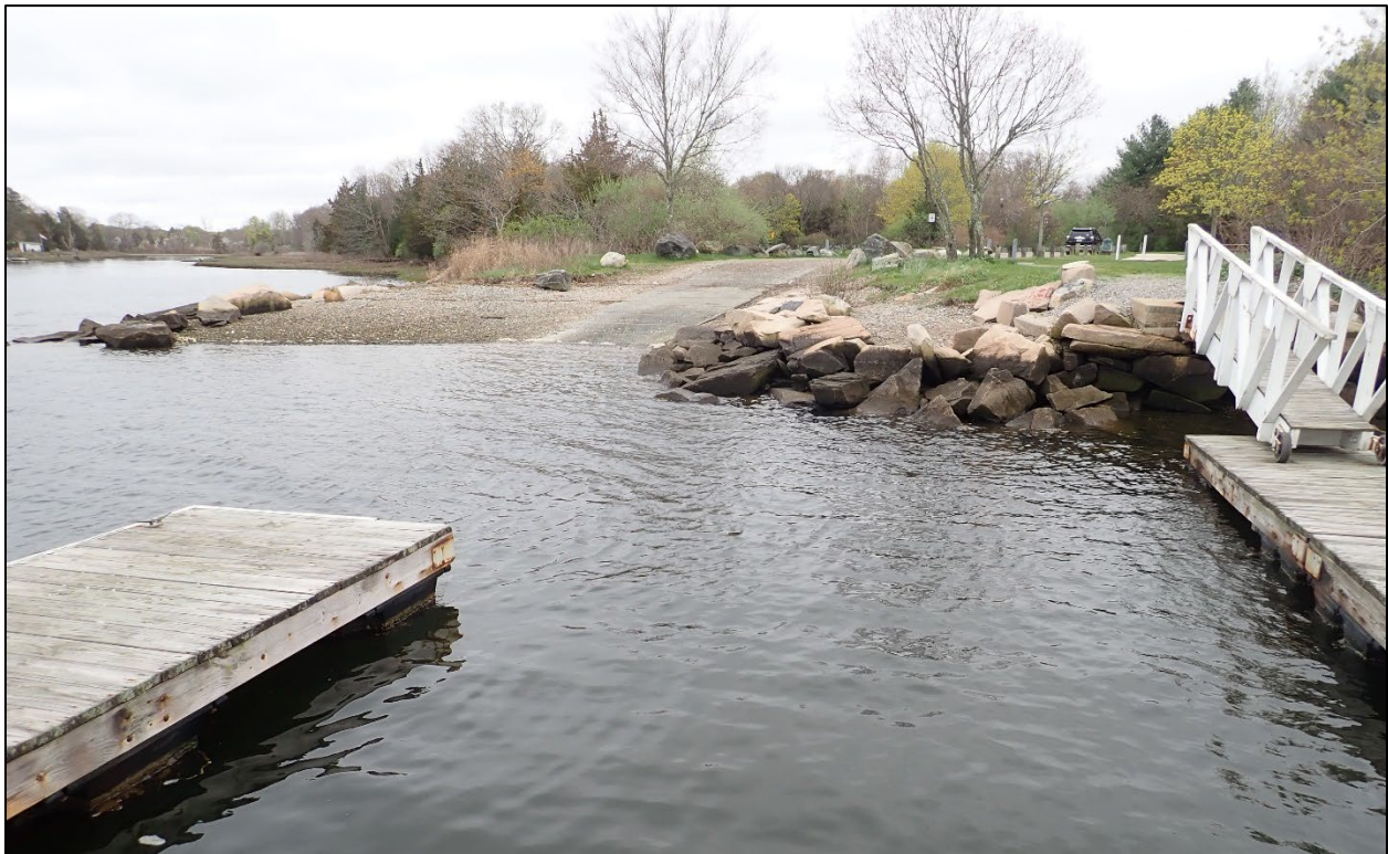
Photo 4: The concrete boat ramp as seen from the associated timber docks.
