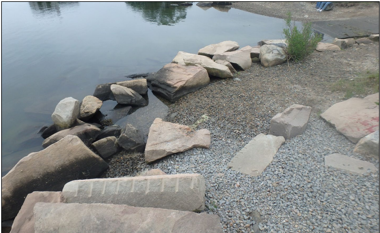
Photo 2: The stone revetment looking south.
