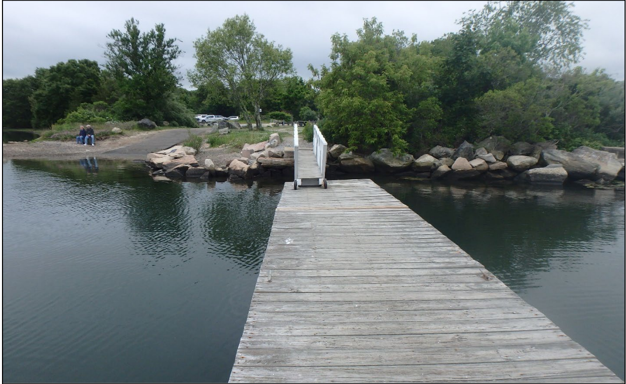
Photo 1: The stone revetment looking southwest.
