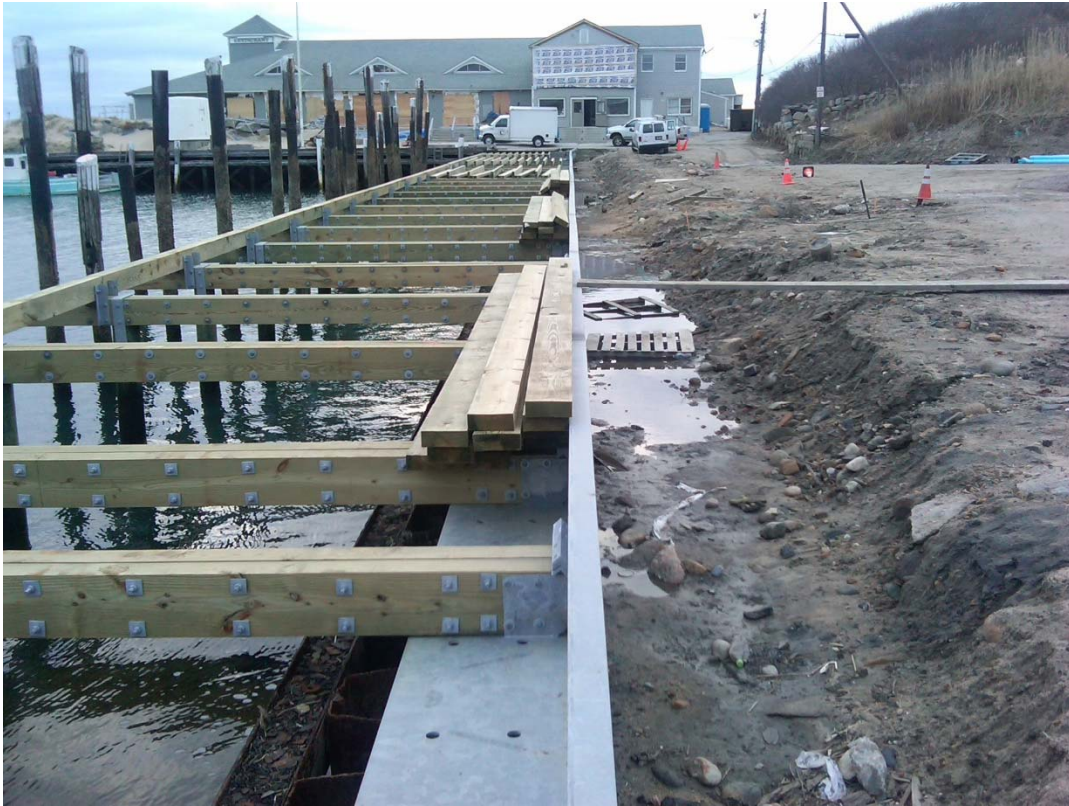
Steel Bulkhead Pile Cap and Start of Timber Framing
