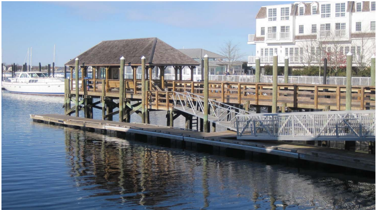
Completed Pier Looking North West
