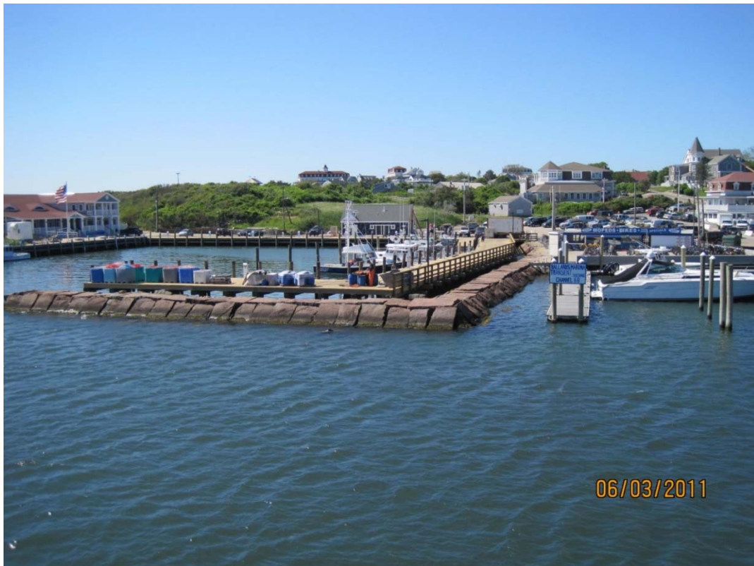
Completed Dock Facility
