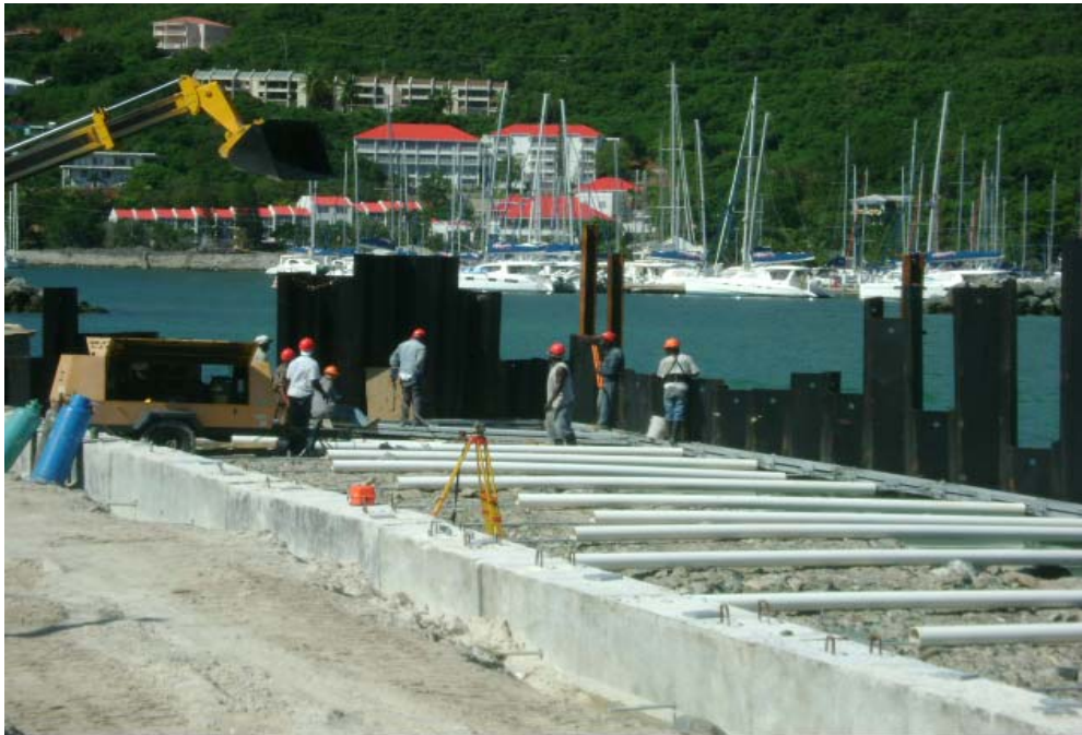
Tender Pier Sheet Pile Wall During Construction
