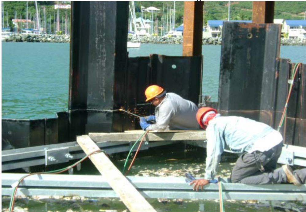
Cutting Sheet Piling to Finish Elevation
