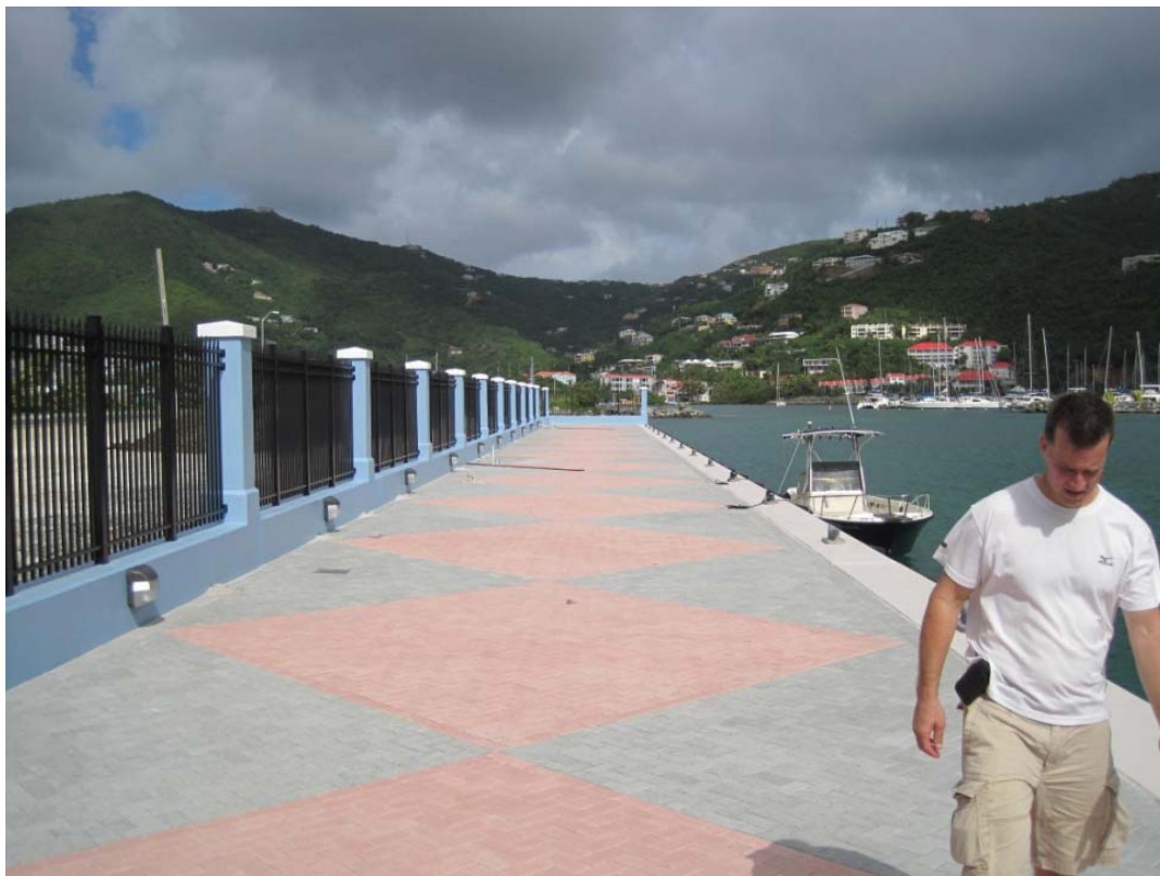
Completed Tender Landing
