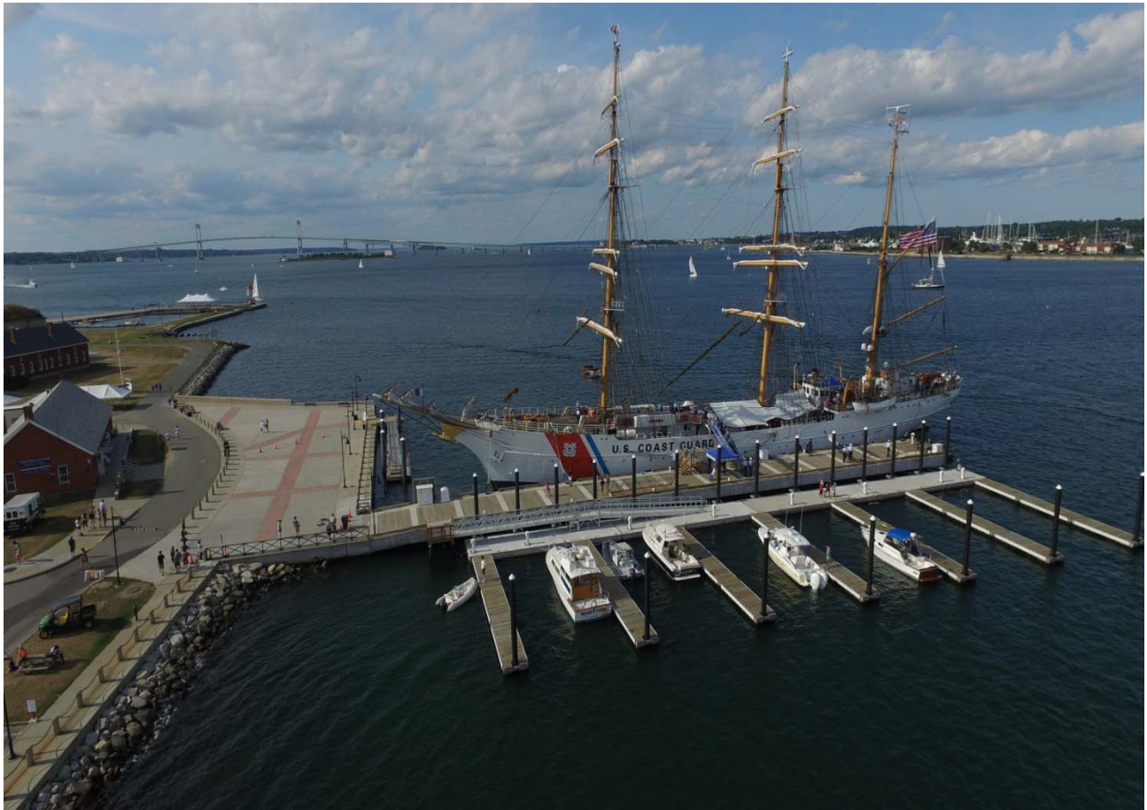
Completed Facility with the U.S. Coast Guard Tall Ship, The Eagle, Berthed Along the North Face of the Pier
