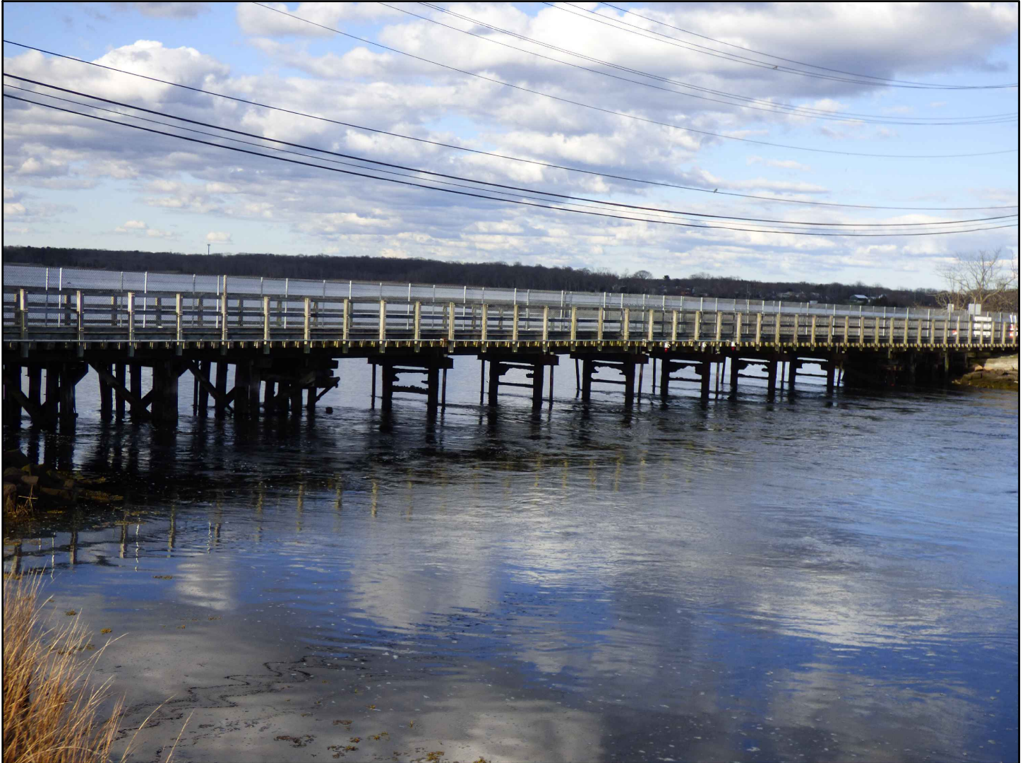
Palmer River Bridge
