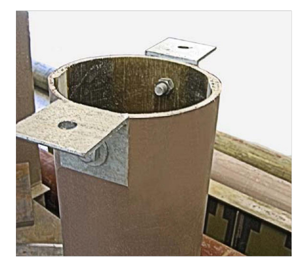
Assembled Brackets - 10" Pile
