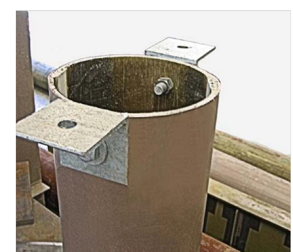
Assembled Brackets - 10" Pile
