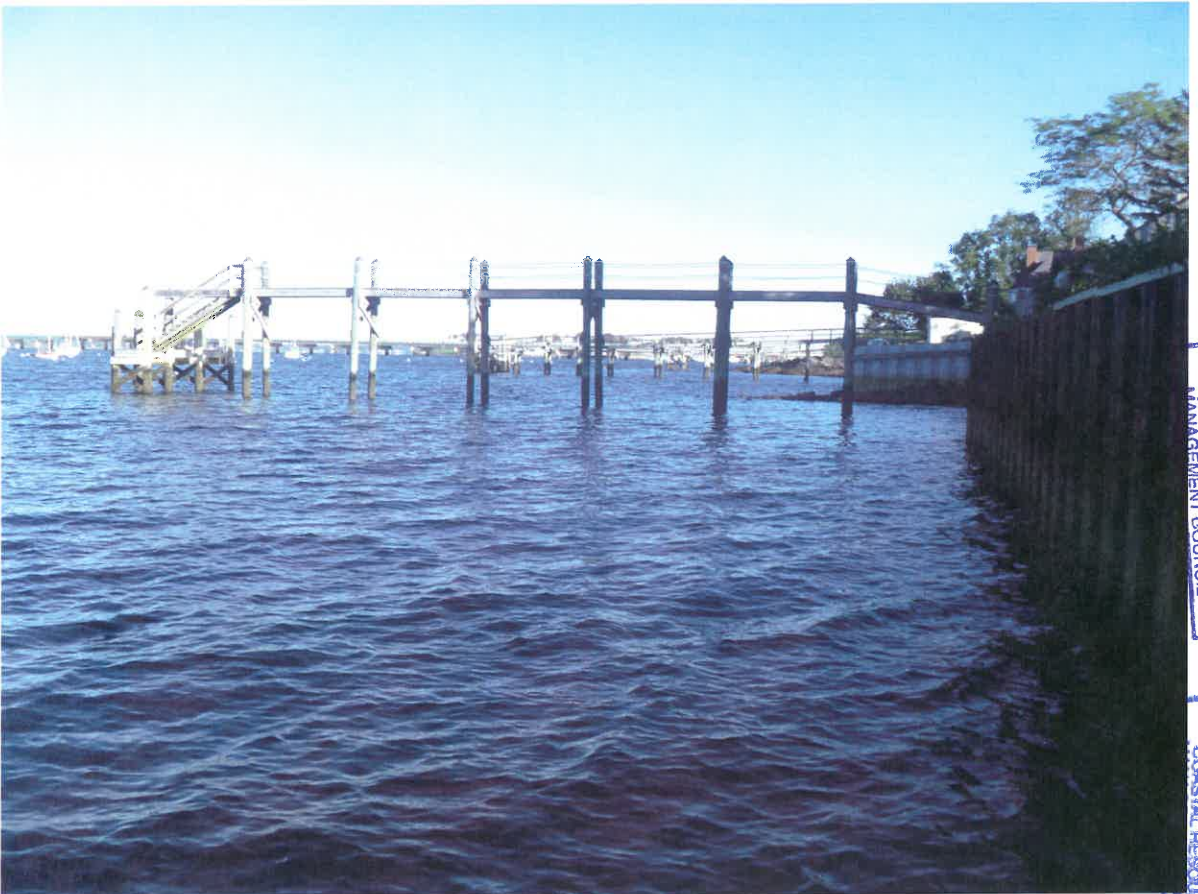
Looking north along applicant's seawall at existing dock to the north.
