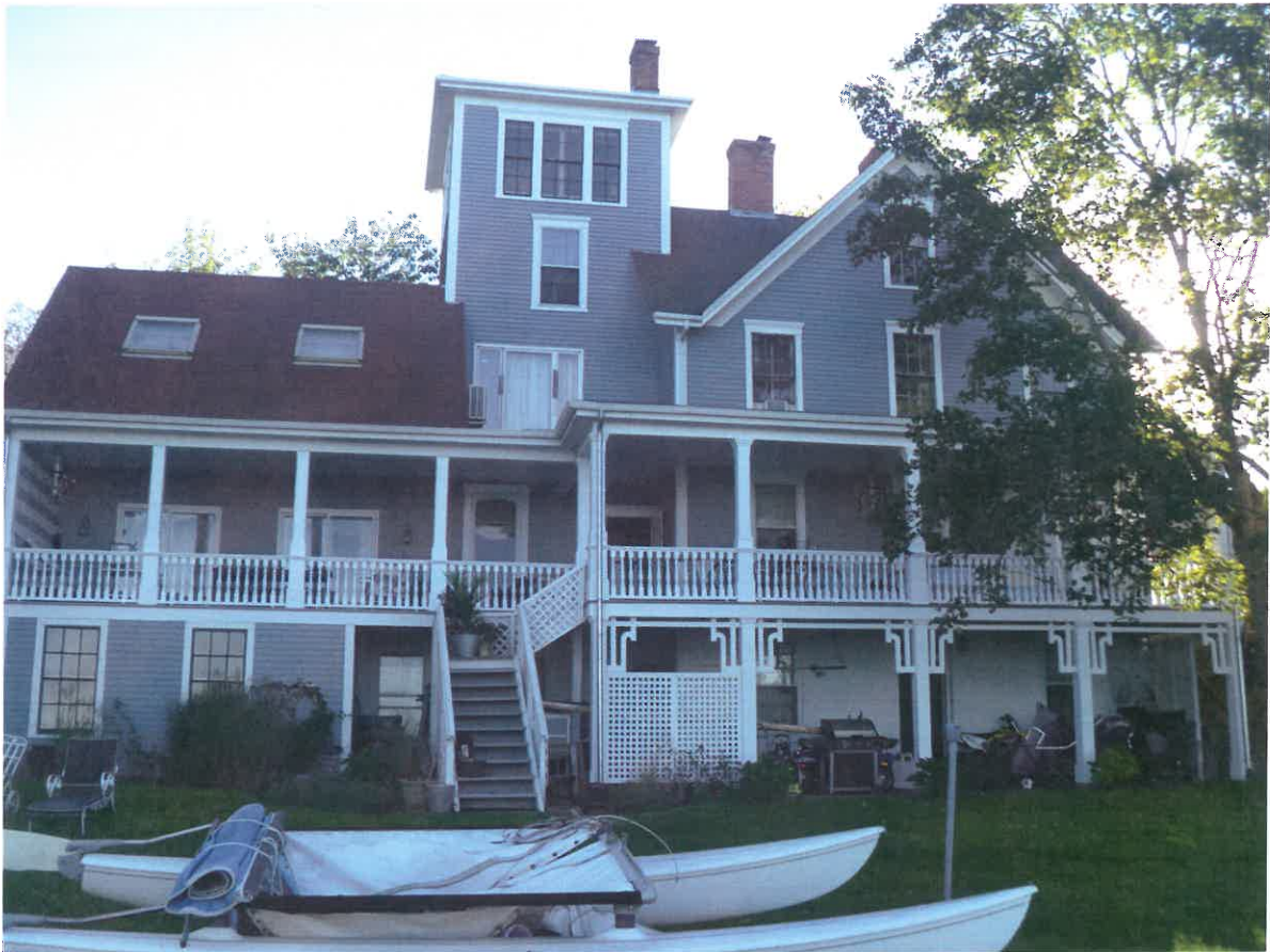
Rear yard of existing house looking east from water.
