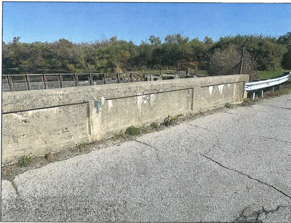
Photo No. 2: View of northern parapet and bridge plaque.
