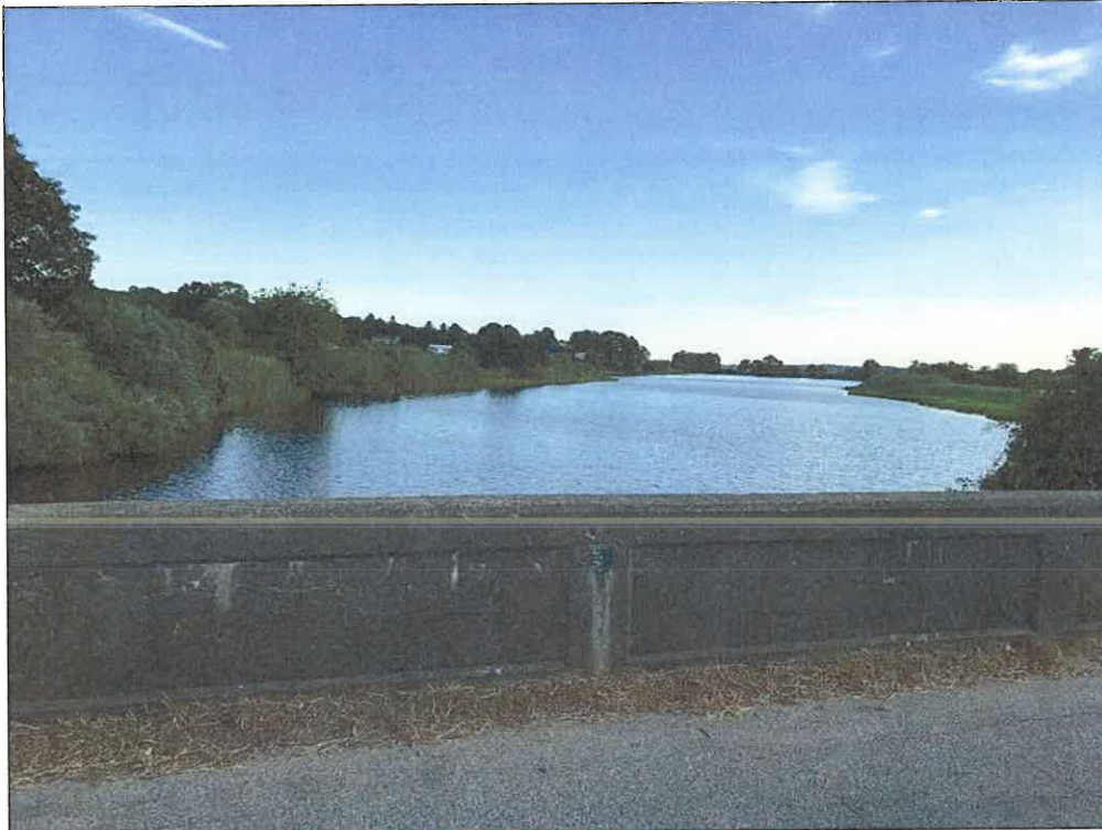
Photo No. 5: Overall view of Almy Creek facing south from the bridge.
