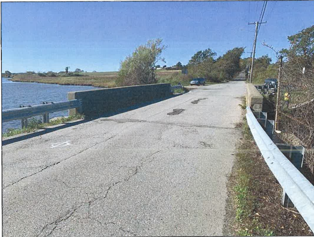
Photo No. 3: View of roadway and bridge facing west.
