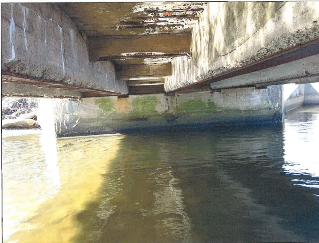
Photo No. 4: Typical view of bridge underside facing west.
