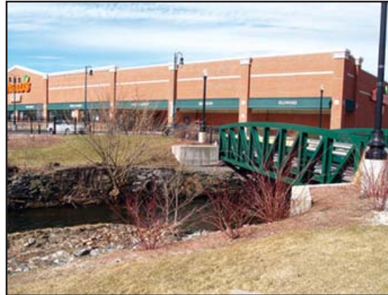
Photo credit: Austin Becker Eagle Square with possible future kayak access
