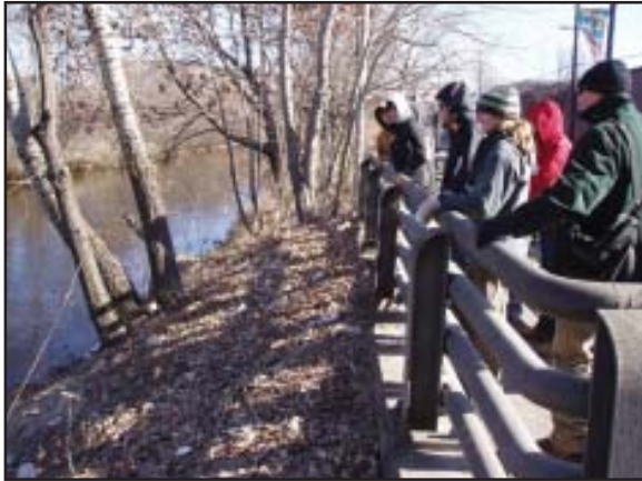
Photo credit: Caitlin Chaffee Metal guard rail
