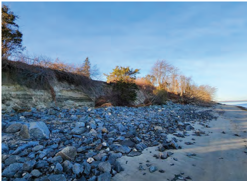
Photo 2. Coastal Features - North. Looking north along shoreline. William Janikies. December 26, 2022.
