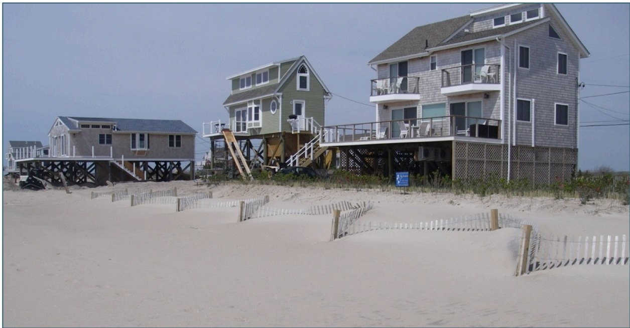
Elevated homes in Westerly, R.I. The green house (center) has been elevated to 5 feet above the base flood elevation.
