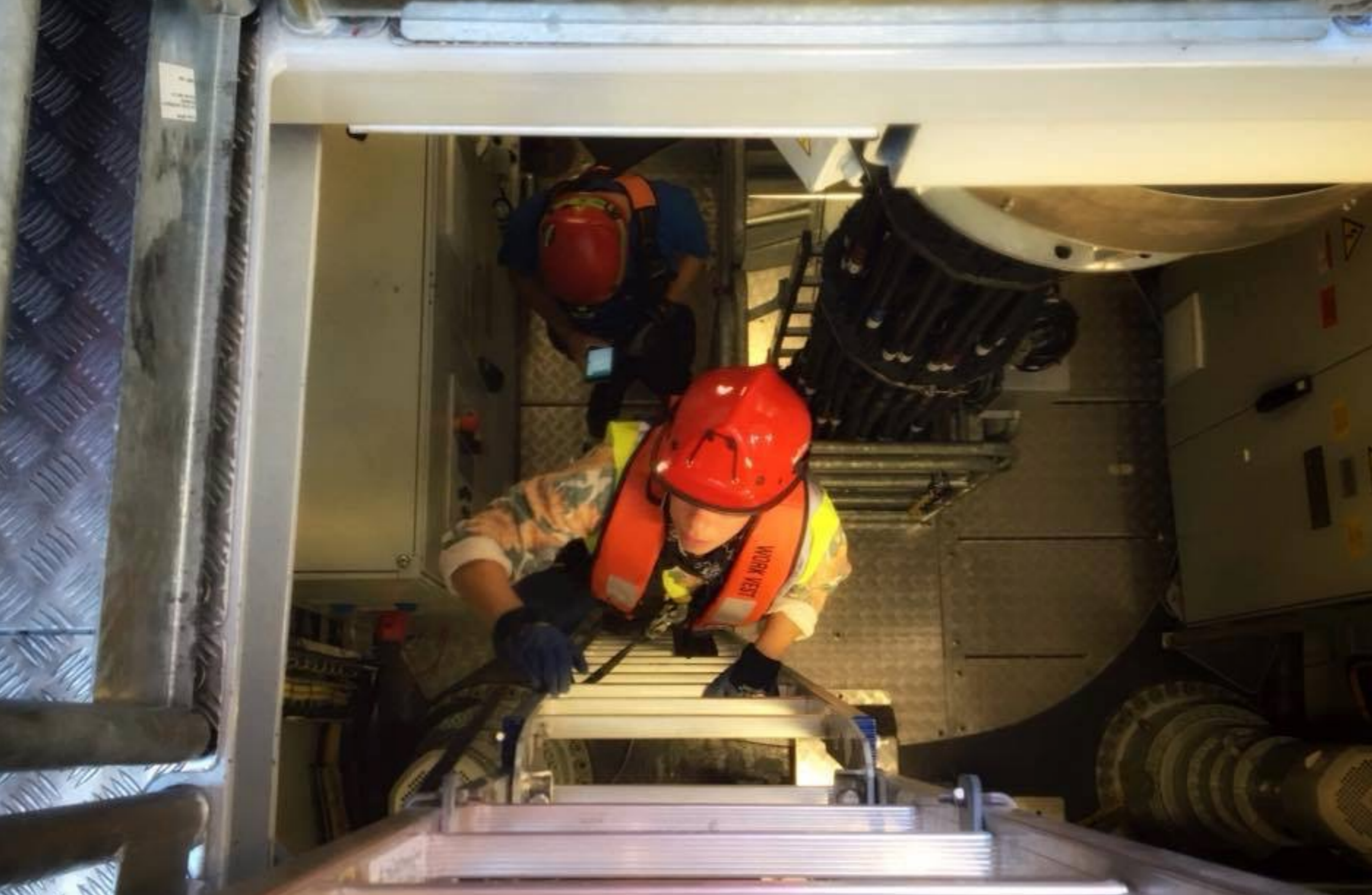
NACELLE INTERIOR- LOWER SECTION
