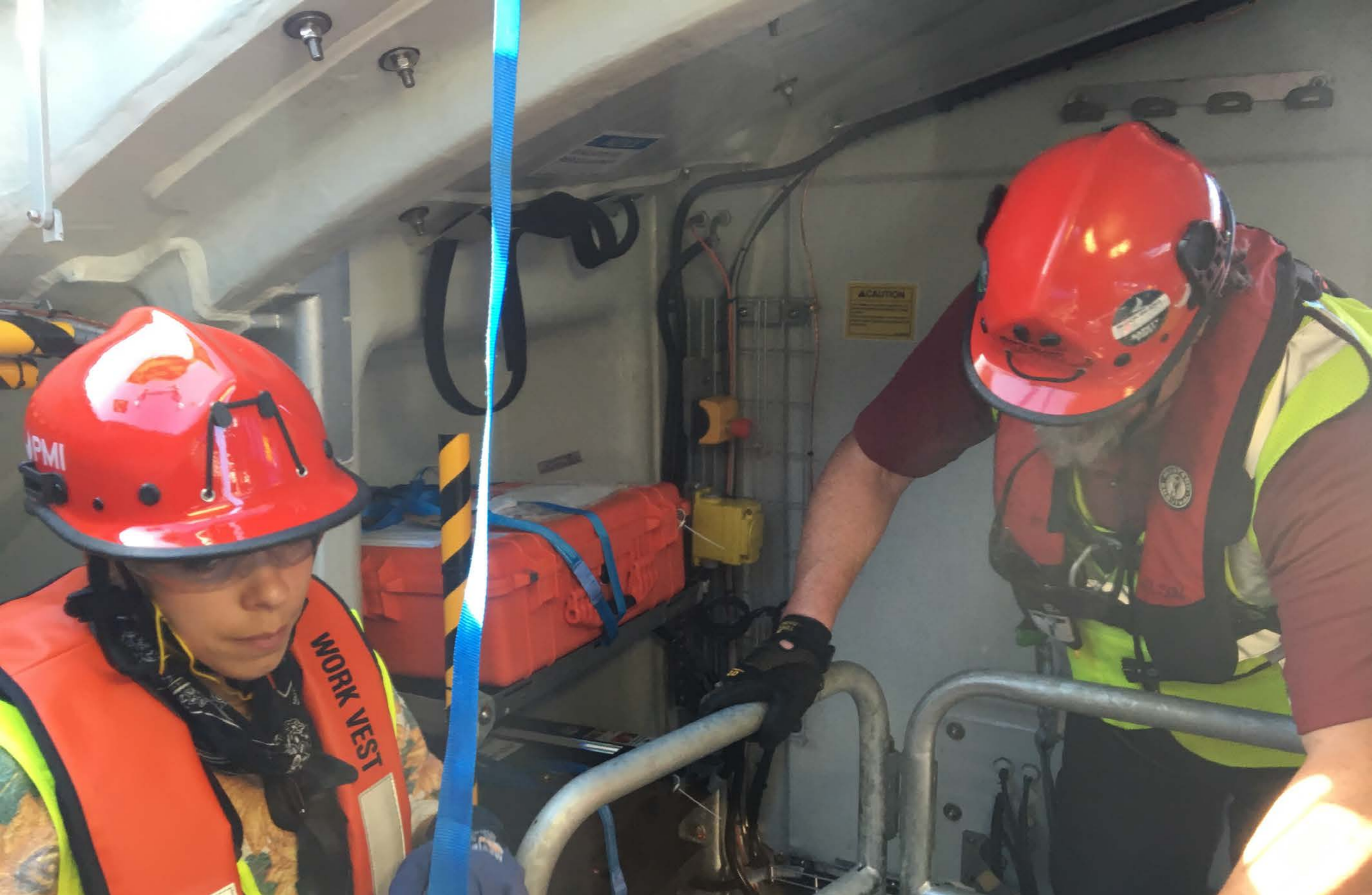
NACELLE INTERIOR- UPPER SECTION
