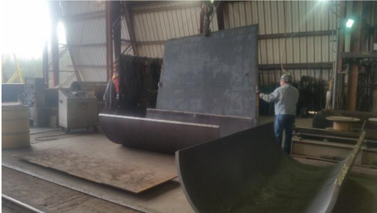
Racetrack connection of Deck – Gulf Island Marine, Houma, LA
