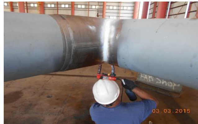
MT performed on the deck X-Braces
