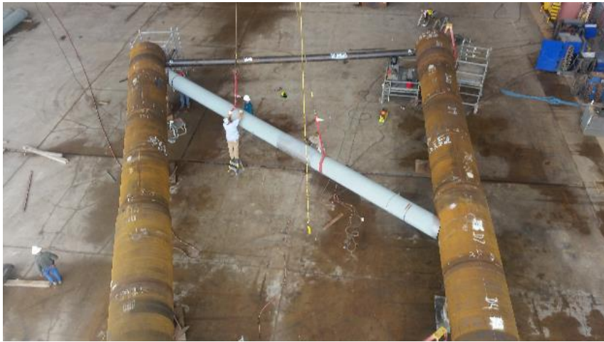
Brace being installed to first two deck legs for site 1
