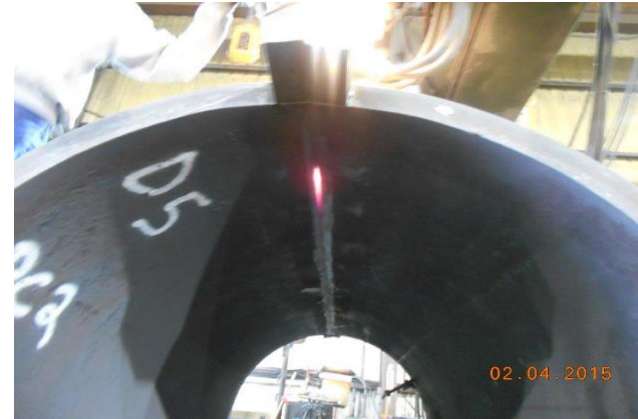
Welding of the 2-1/2" thick can
