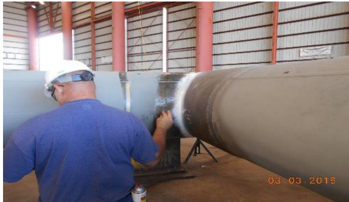
UT performed on deck X-braces
