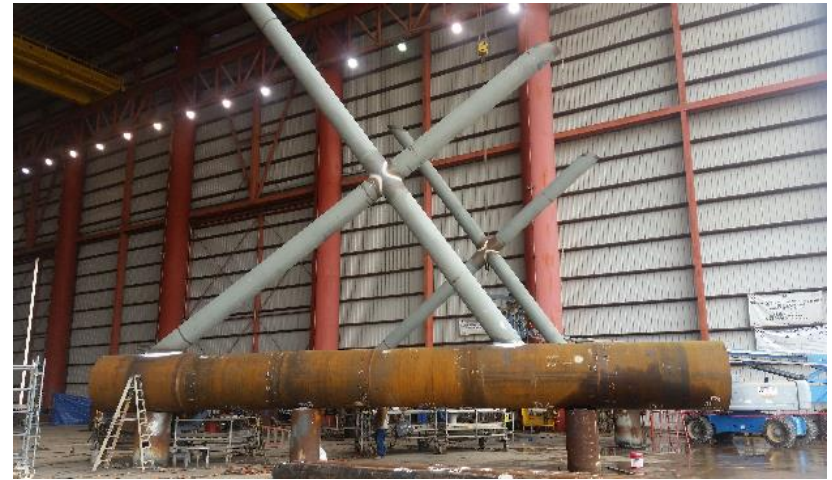
36" X-Braces installed to leg A1 and A2
