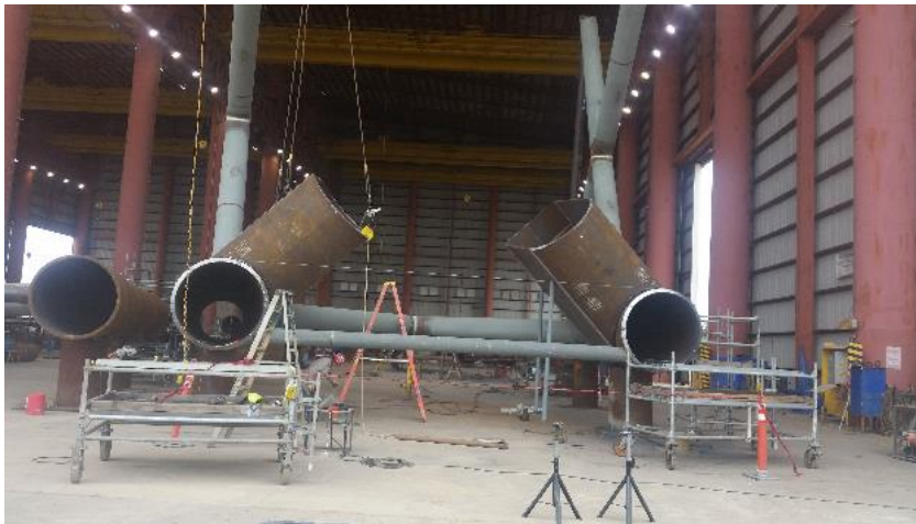
Race track braces being prepared to be welded
