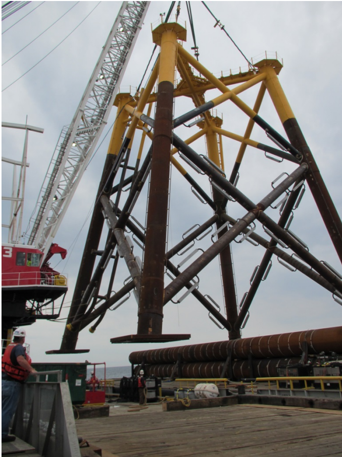
Jacket 1 – Lift from Cargo Barge
