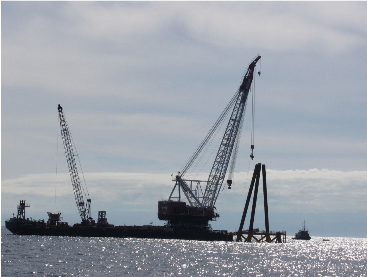
Jacket 3 – 3 of 4 P1 Piles Stabbed
