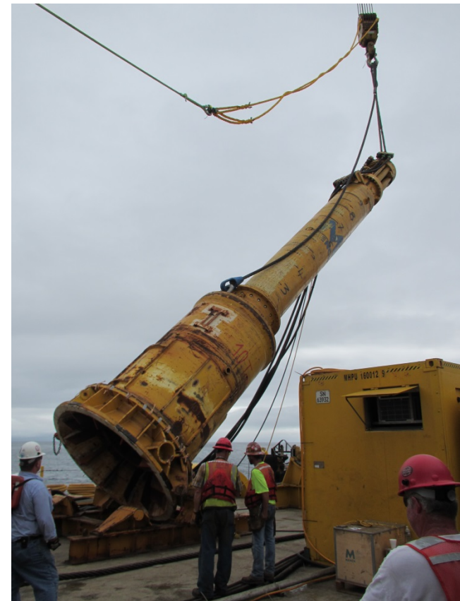
Pile Driving Hammer
