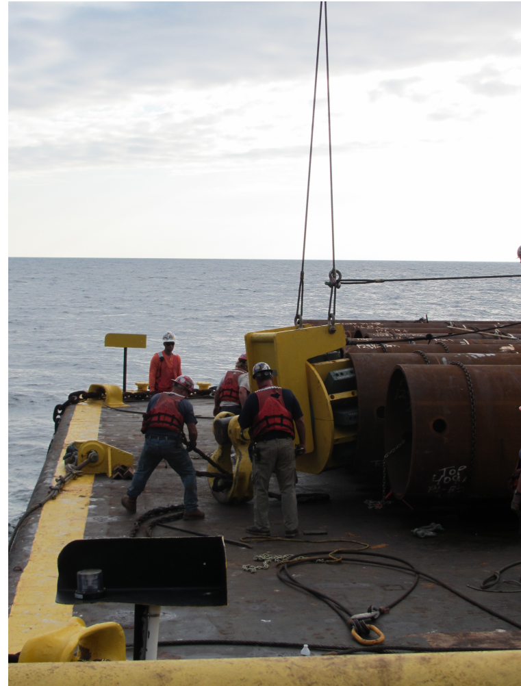
Rigging of P1 Piles
