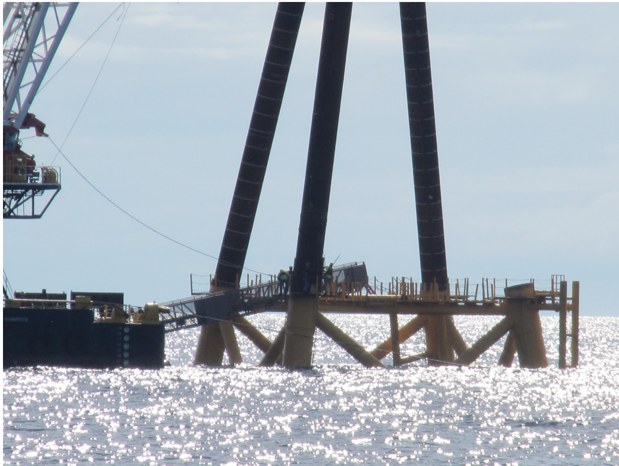
Installation of 3 rd P1 Pile Jacket 3
