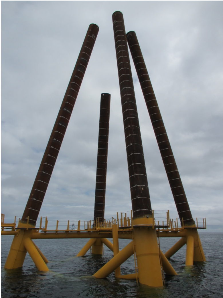
Jacket 2 – P1 Piles Stabbed
