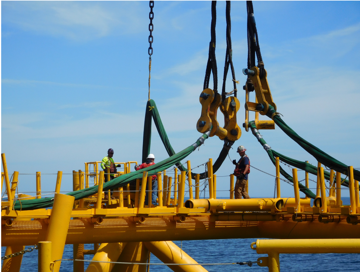
Rigging for Jacket Lift
