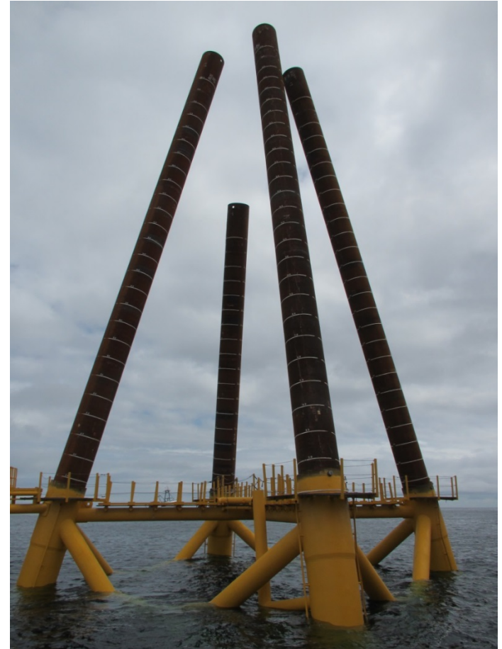
P1 Piles Stabbed
