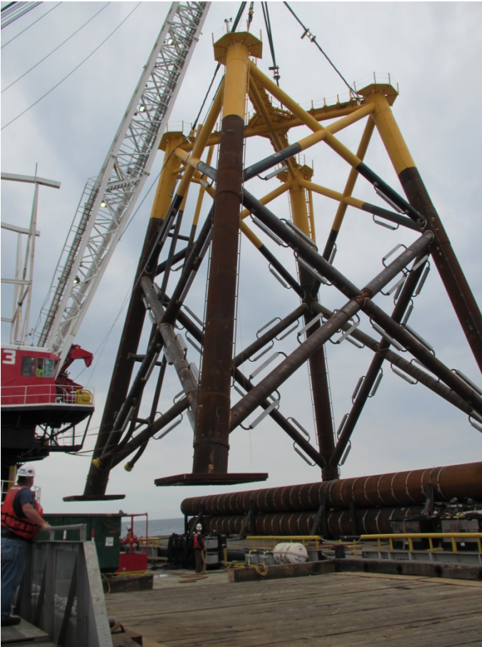
Jacket Lift from Cargo Barge
