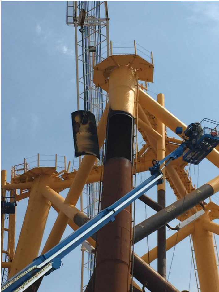
Jacket 1 Repair in Progress
