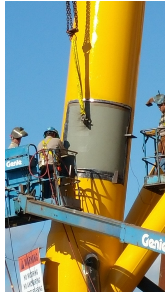
Deck 2 Repair in Progress
