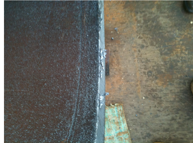
Jacket 1 P1 2 ½ in to 1 ¾ in transition visible on cut off section
