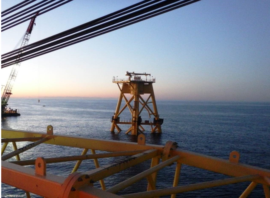
Deck 1 Set and Levelled Nov 2
