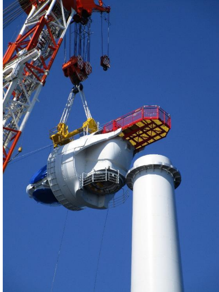
RNA Lifting and Setting
