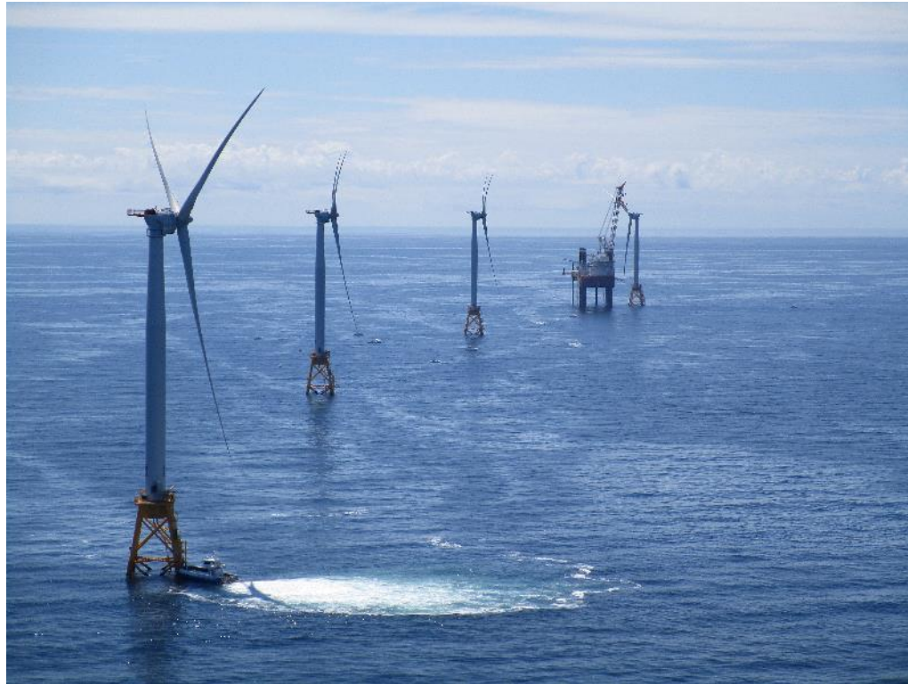
Installation at BI5 and Personnel Transfer at BI2 – from BI1
