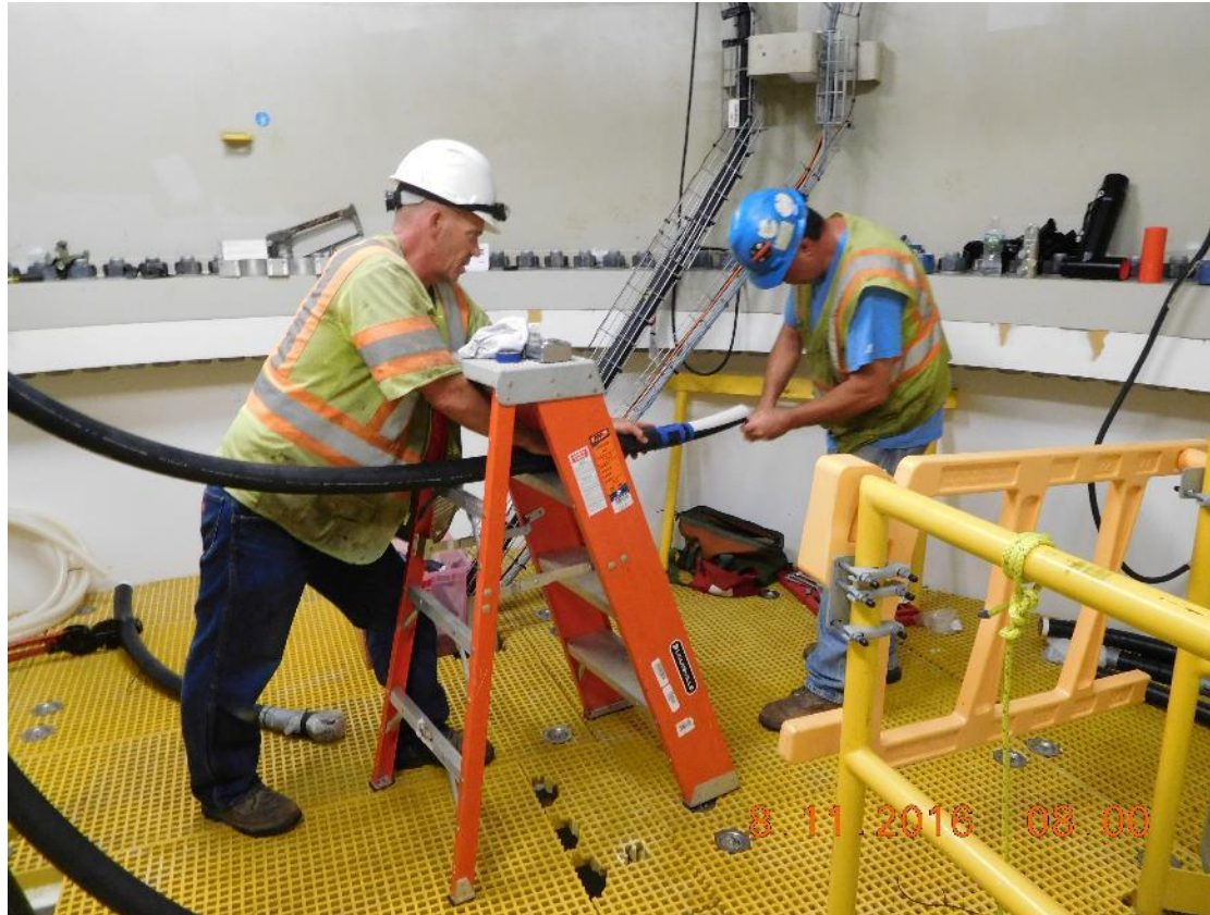
Routing and Terminating HV Cables
