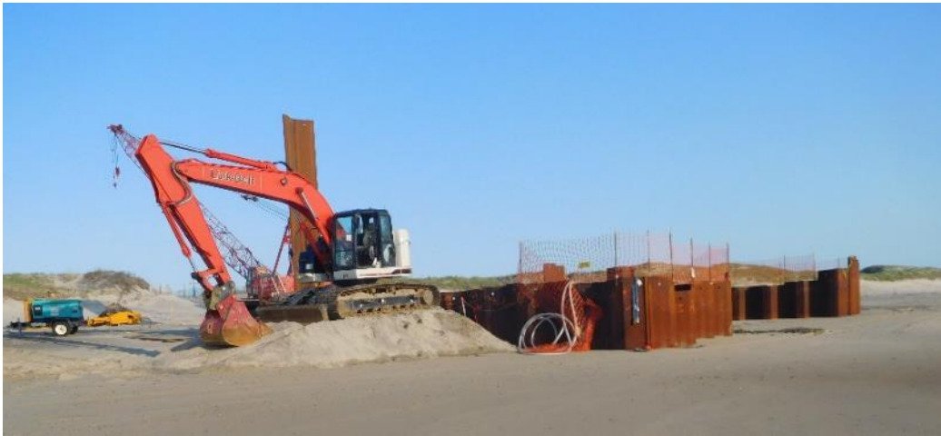
Coffer Dam on Crescent Beach
