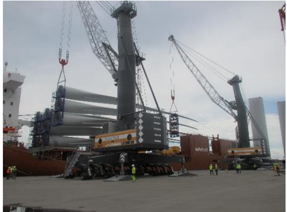
Offloading blade assembly 1 with ProvPort cranes
