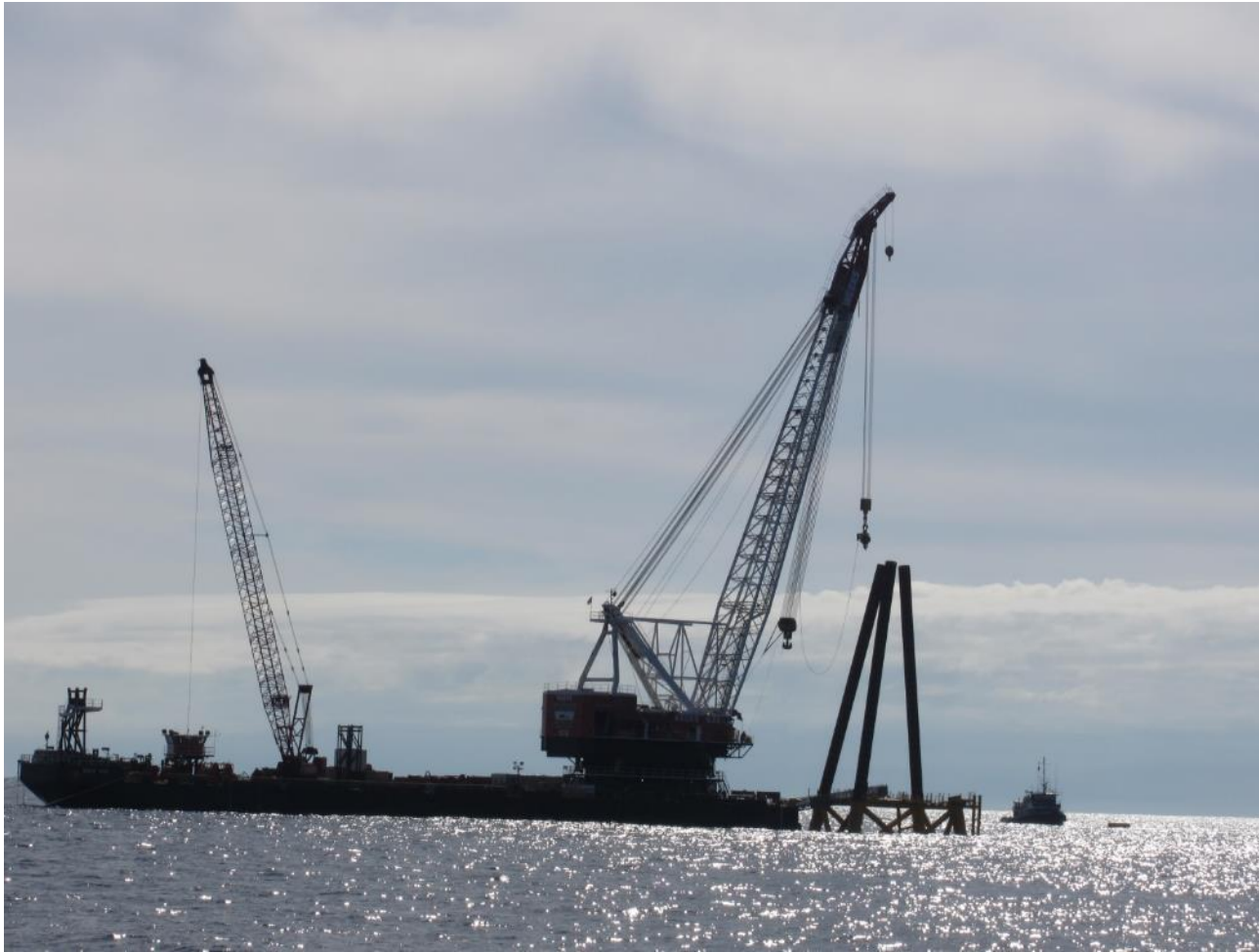
Pile Stabbing and Driving with W533
