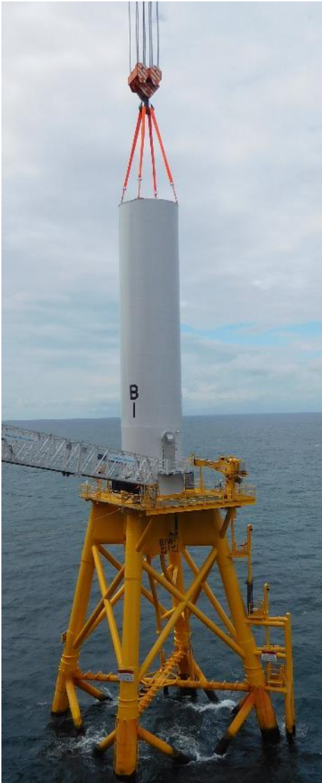
Tower Lifting and Setting
