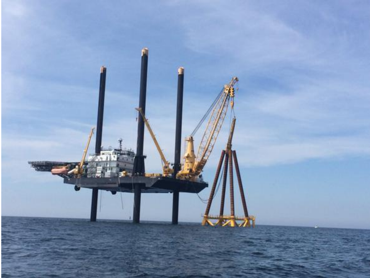
Pile Stabbing and Driving with Lift Boat Robert
