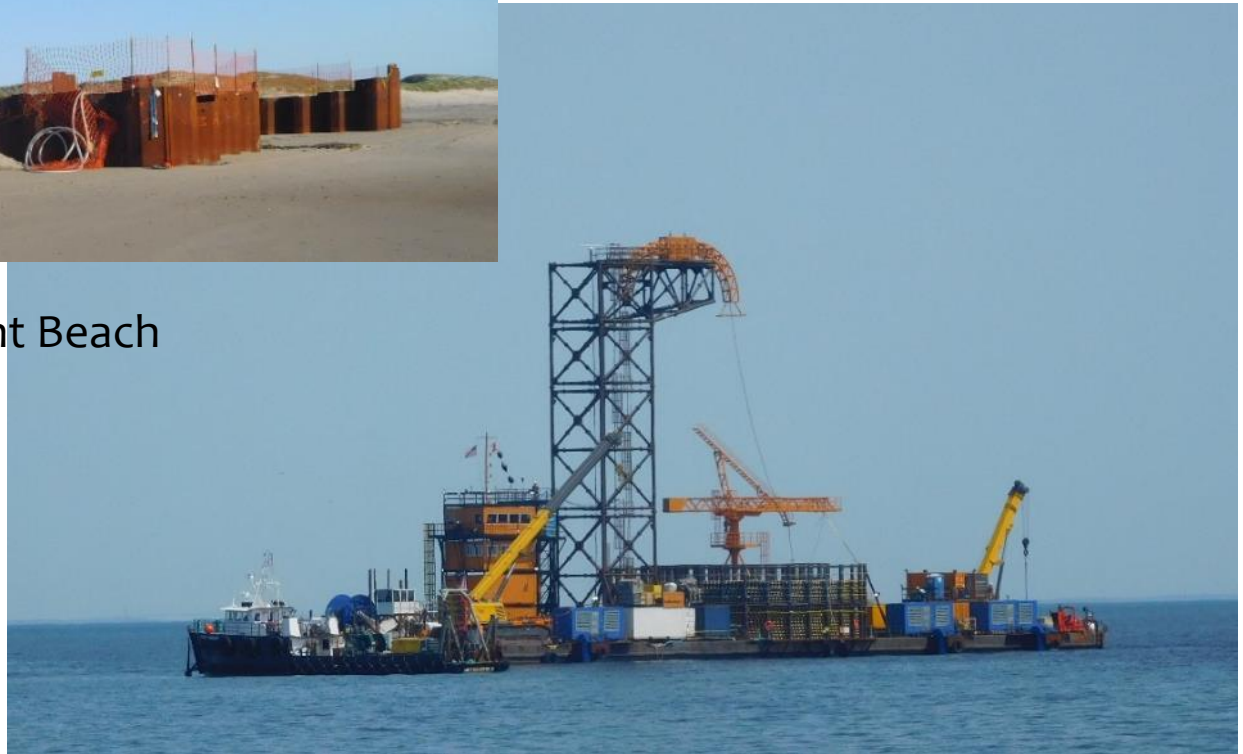
“Big Max” Cable Lay Barge
