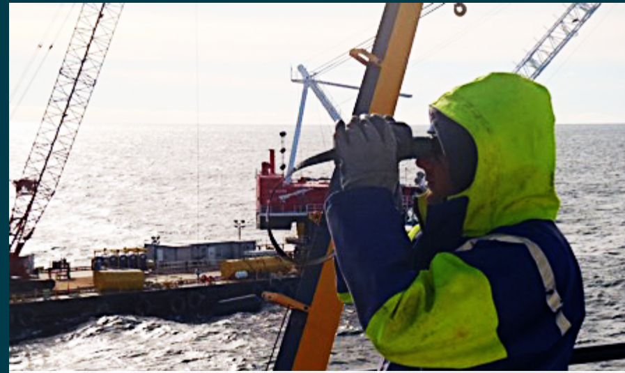
Protected Species Observer (PSO) Block Island Wind Farm Foundation Installation
