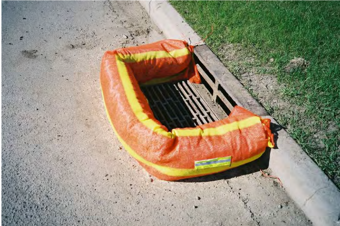
Curb Inlet or Drop Inlet Catch Basin Protection 06/2021 N.T.S. Source: VHB
