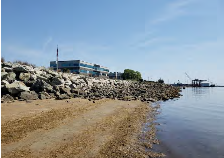
Photo 1: Coastal beach at the landfall work area. The riprap shoreline protection is placed in front of a cast in place seawall at the landward side of the revetment and forms the Shoreline Feature. Photo date: May 20, 2021
